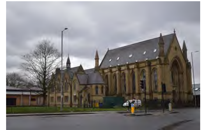
3.37 Railings and gates to the west
