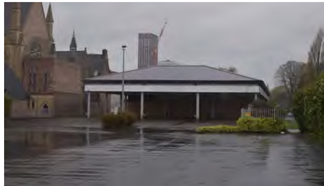
3.41 Former dealership to the east
