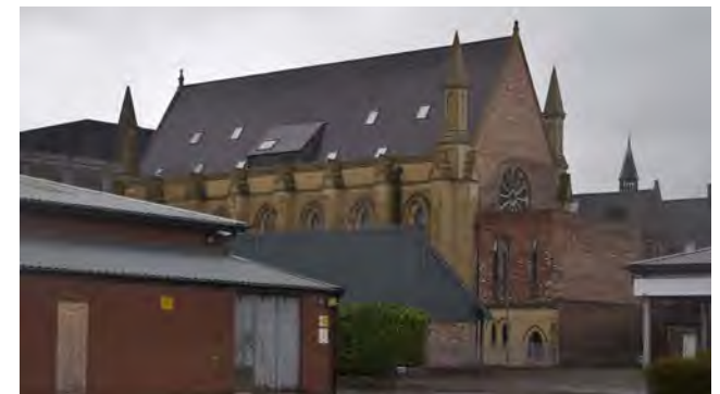
3.45 South elevation, with extension to the chancel
