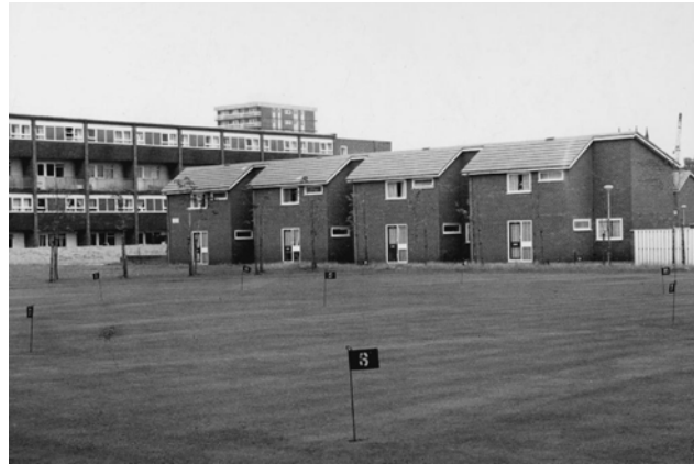
2.15 Brunswick Estate, showing new housing to the rear of Kincardine Road putting green, 1970 (Local Image Collection)
