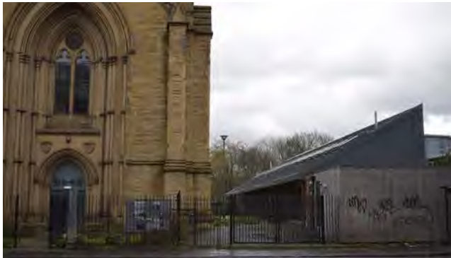
3.38 Railings and gates to the west
