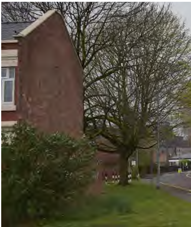
3.33 Northeast flank wall
