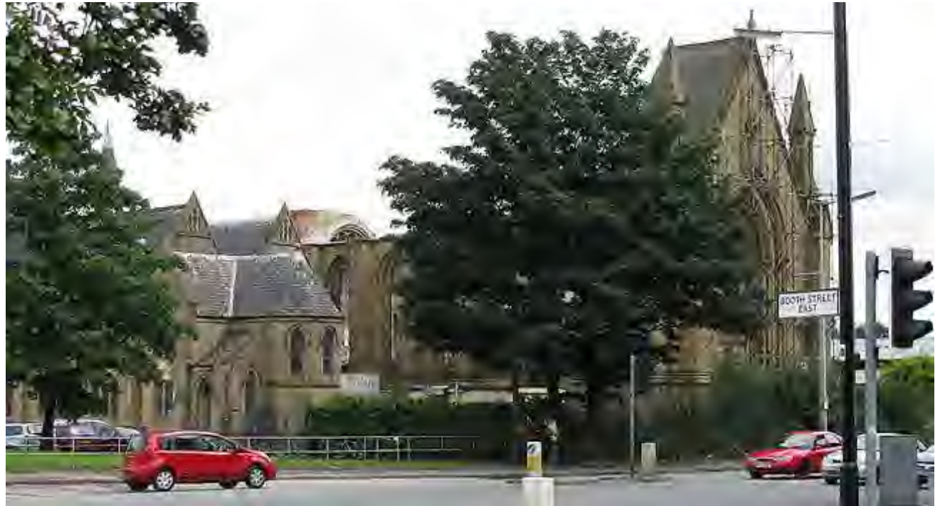
2.26 Former Unitarian Chapel, 2009 (Manchester History)
