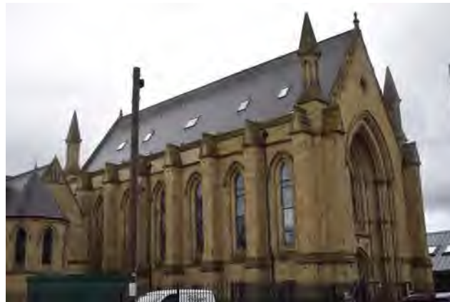
3.46 Roof to the north elevation
