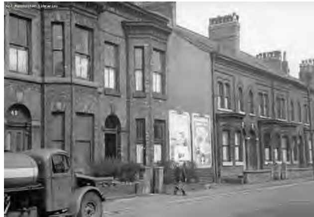
2.9 48-40 Brunswick Street (north side), 1961 (Local Image Collection)
