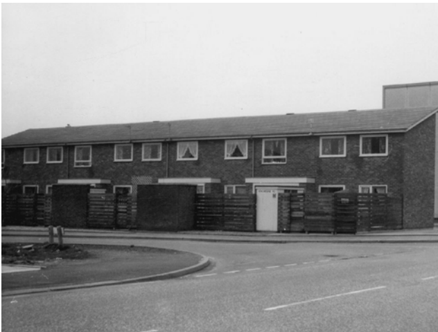
2.14 Brunswick Estate, new housing on Kincardine Road, viewed from Brunswick Street, 1972 (Local Image Collection)
