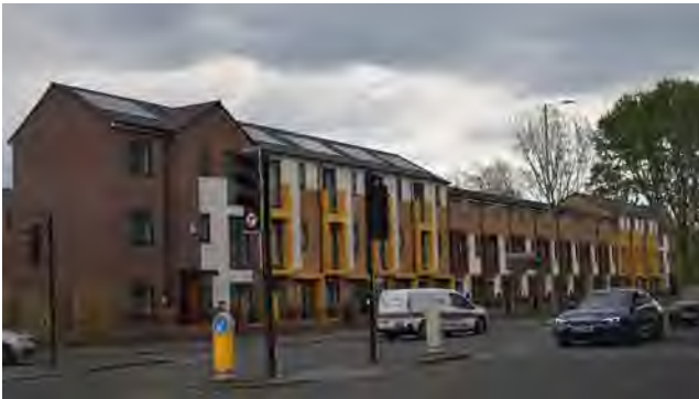
3.13 Townhouses to Upper Brook Street
