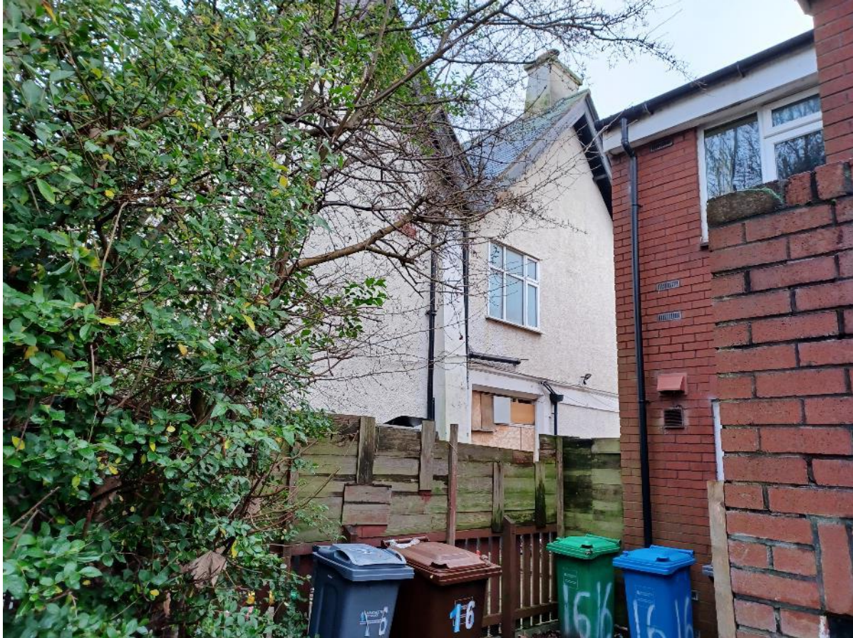
View from 14-16 Mobberley Close towards the Former Pub building
