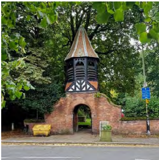
Figure 3: Lych Gate at present.
