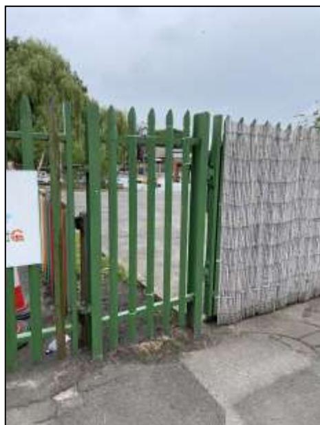
Photograph 4 – Existing steel palisade fencing enclosing the Nursery playground on Chepstow Road
