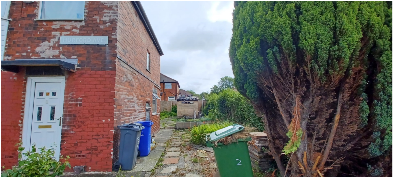
Figure 2. View along the side of the property.
