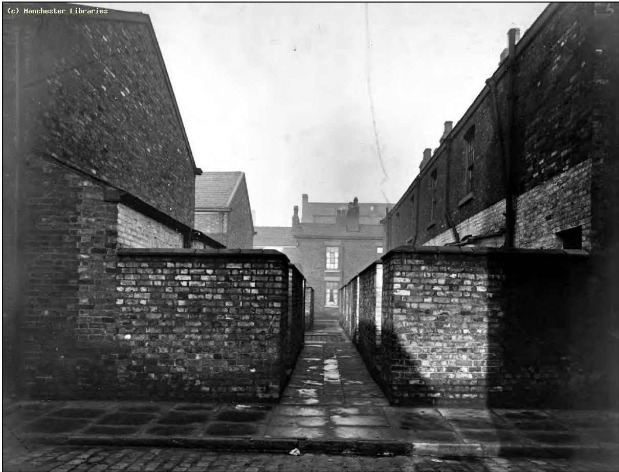
Plate 7 Photograph of no. 24 Wood Street taken from Crown Street in 1900, courtesy of the Manchester local image collection.
