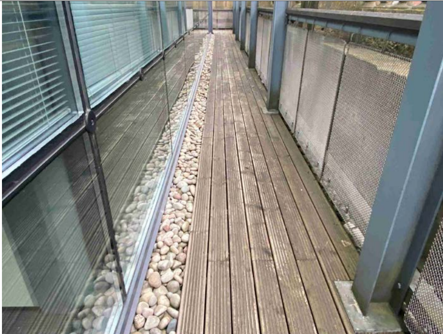
27: Fifth floor balcony walkway
