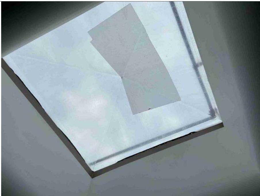
20: Repair to polycarbonate rooflight
