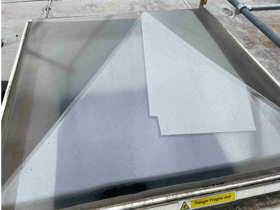
19: Repair to polycarbonate rooflight
