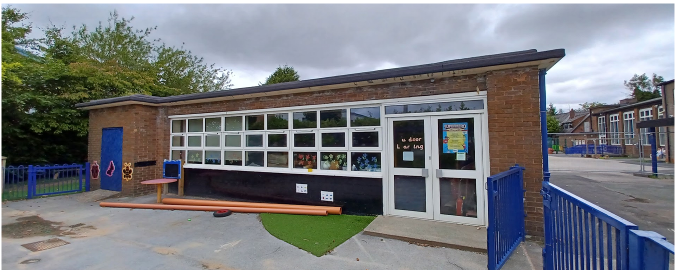
Figure 3. Building to be demolished.
