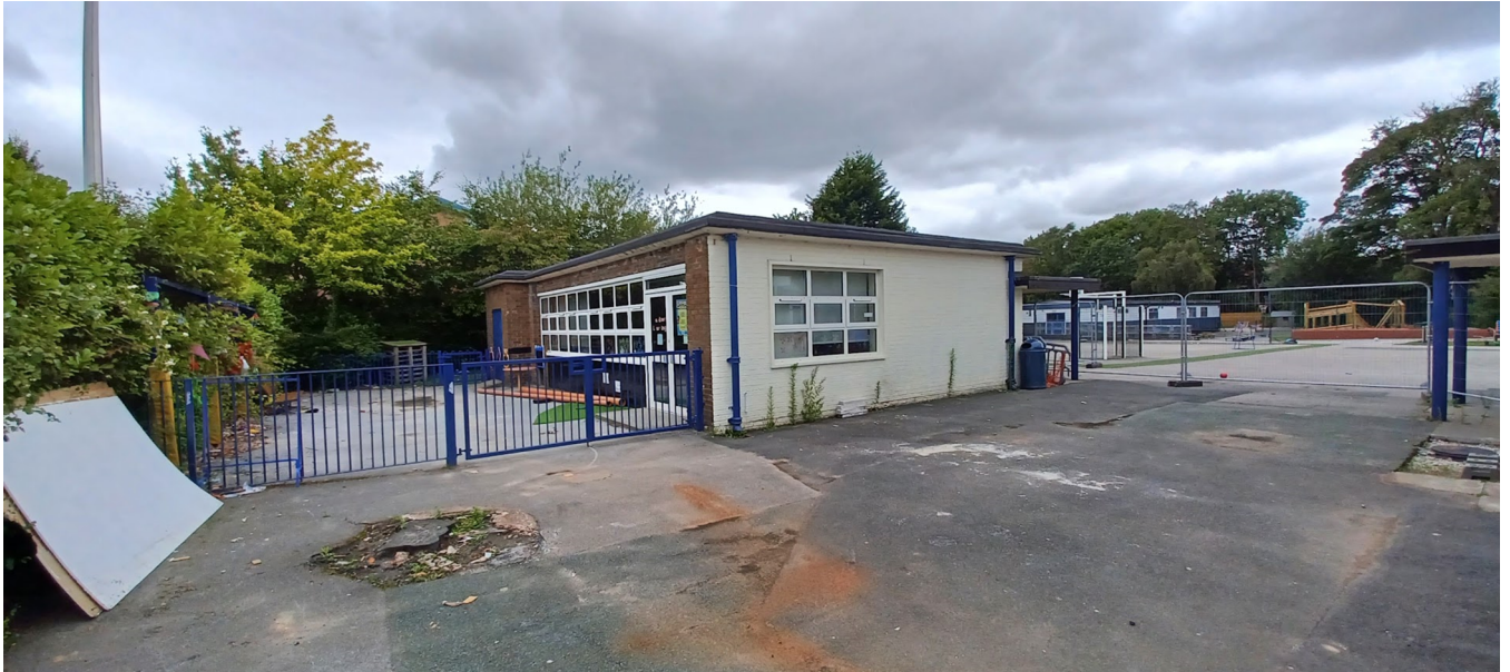
Figure 1. Building to be demolished.
