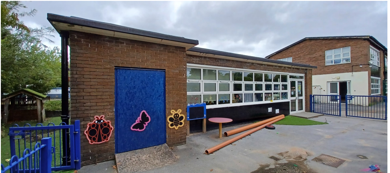
Figure 2. Building to be demolished.
