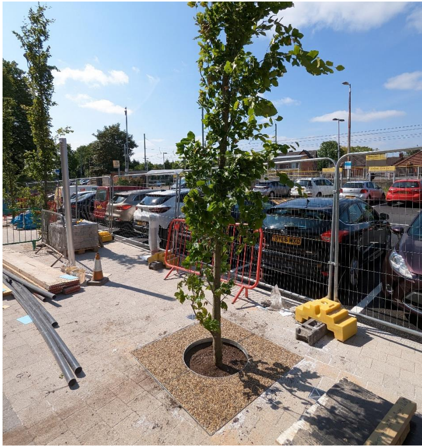
View of the installed tree with underground rooting system along the south-western site perimeter.
