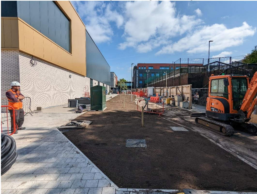
View of the strip of soft landscaping along the south-eastern perimeter of the new building.
