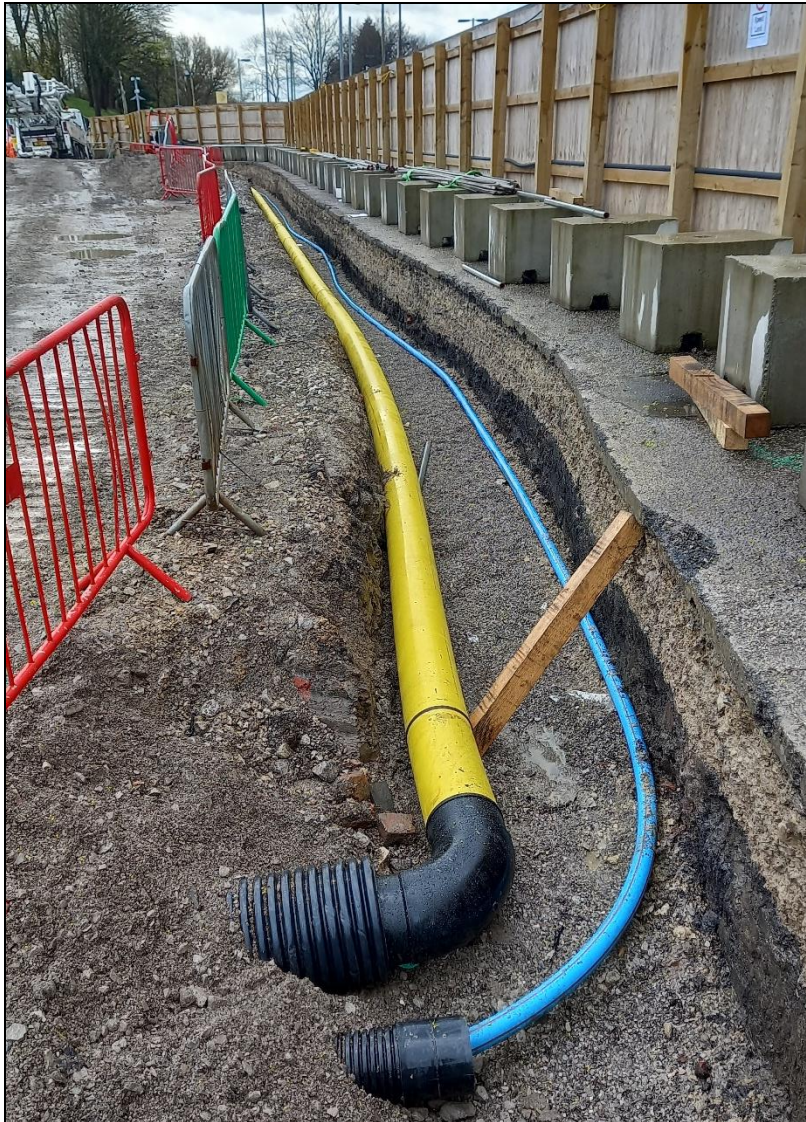
Photograph showing the laid down Puriton® Barrier Pipe (blue) and the gas pipe (yellow) along the south-western site boundary. Photograph taken facing the south-east.
