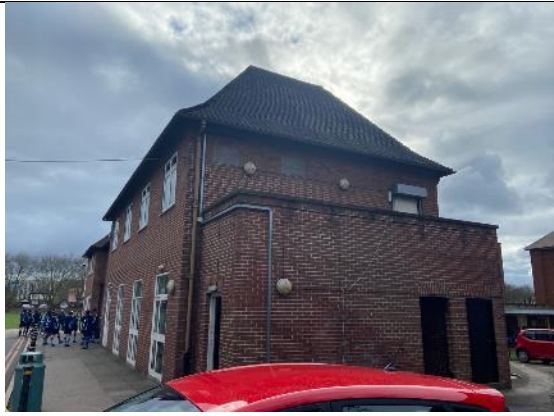
View of the north and east elevations of the pavilion illustrating the bellcast/ sprocketed eaves of the roof which emulate the roof form of the main school buildings. Note modern windows and doors.
