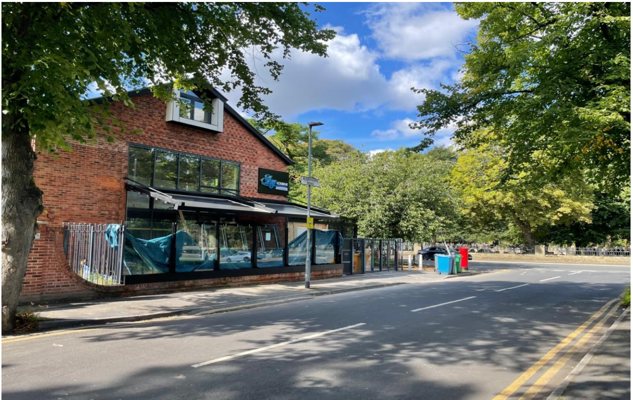
Image 6 – Photograph from Aldermay Road (August 2023) showing site under construction
