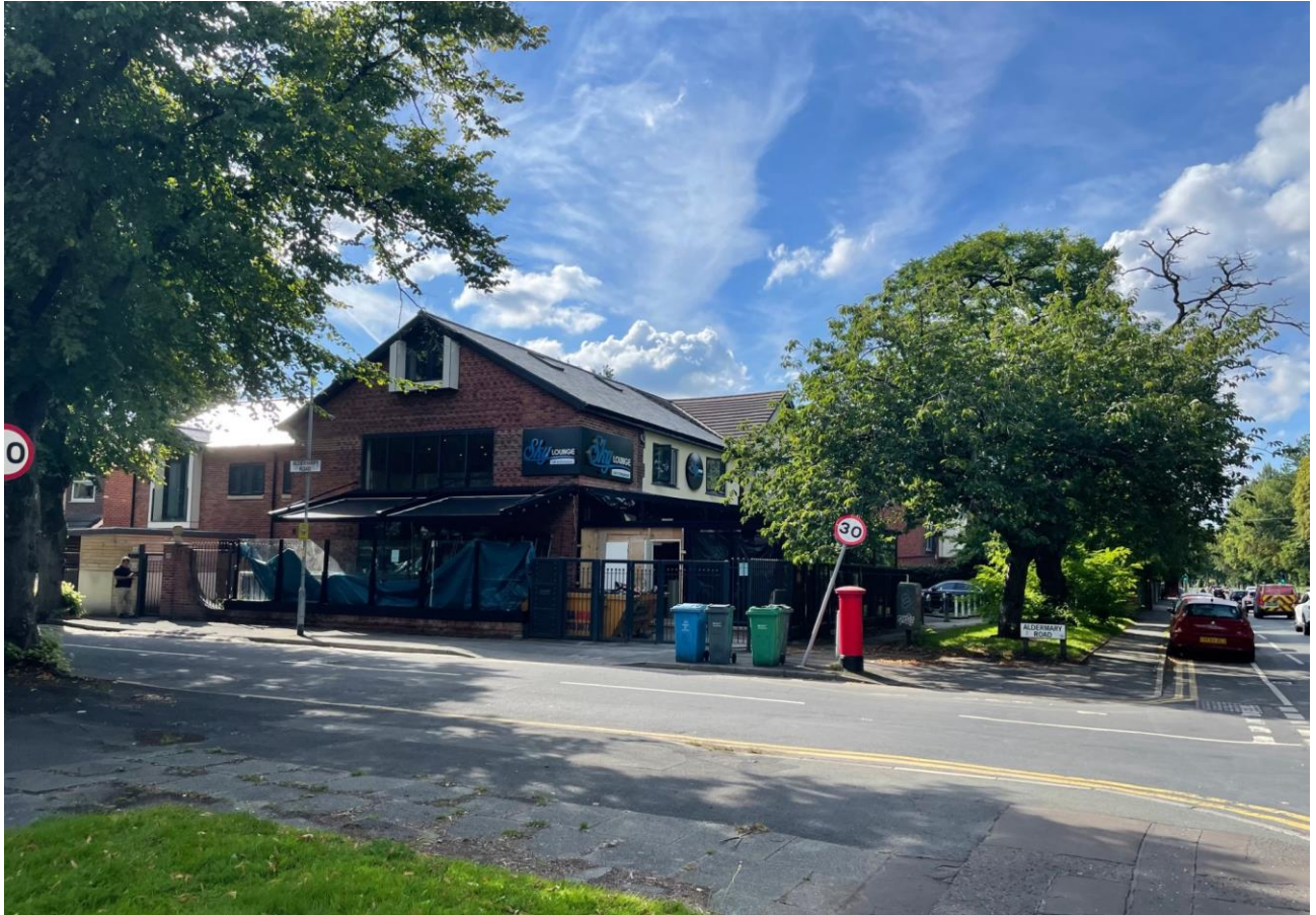
Image 5 – Photograph from August 2023 taken from Barlow Moor Road showing site under construction
