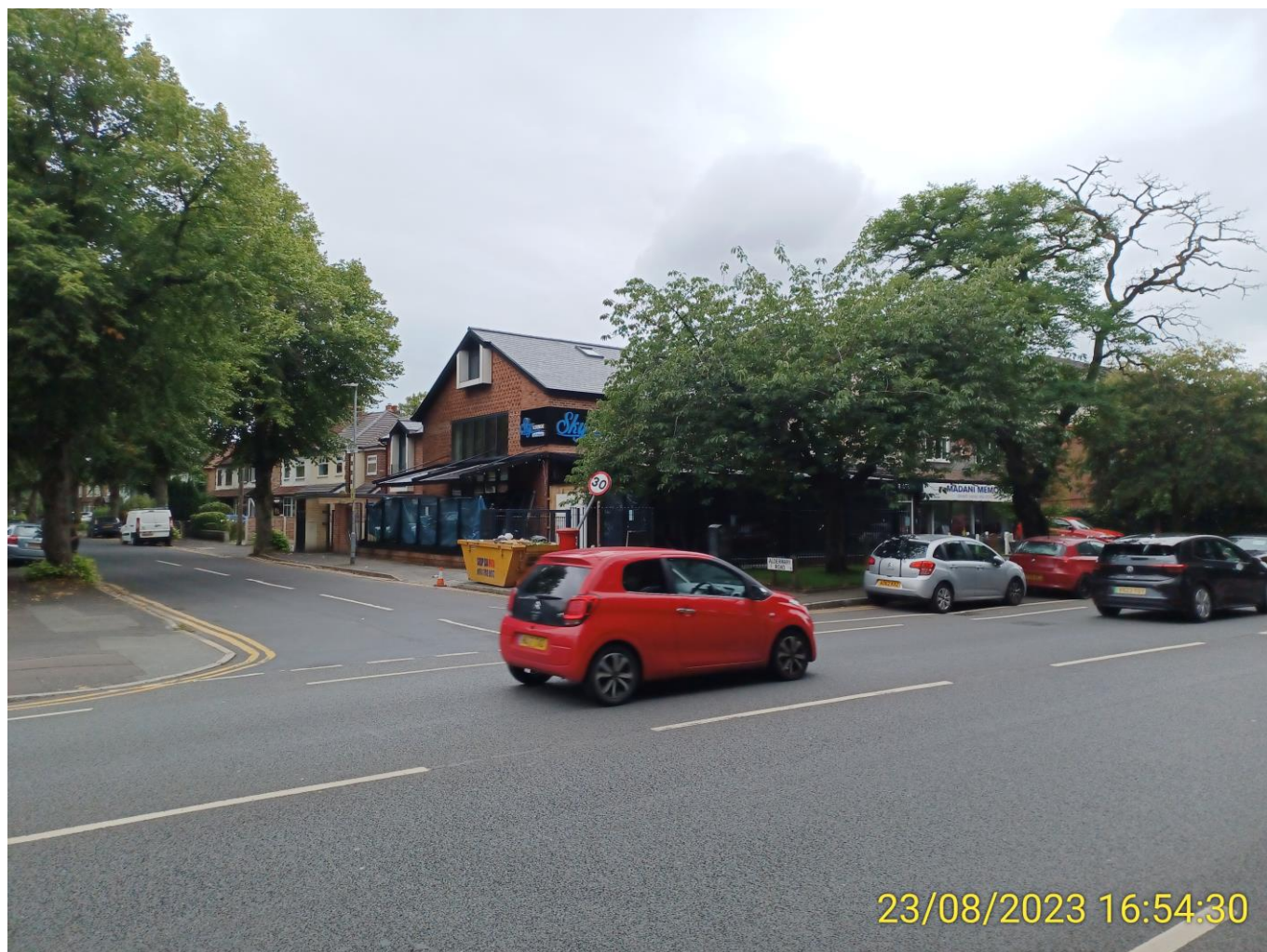
Photograph 1 Application site as viewed from Barlow Moor Road showing both the front and side elevations
