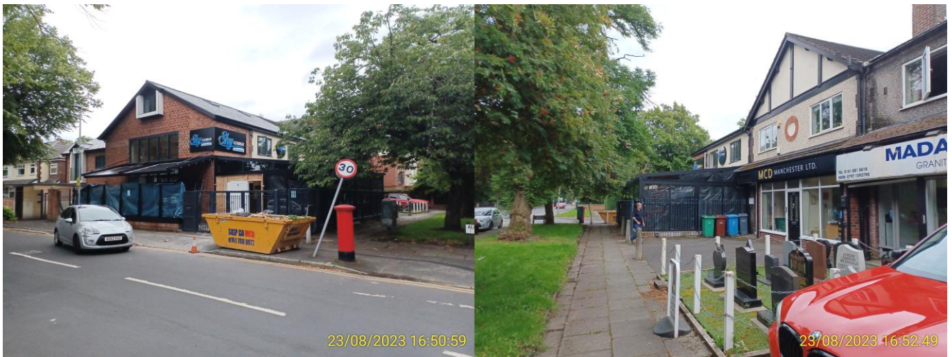
Photograph 2 and 3 Front Extension under construction photographs as dated source: Case Officer Site Photographs
