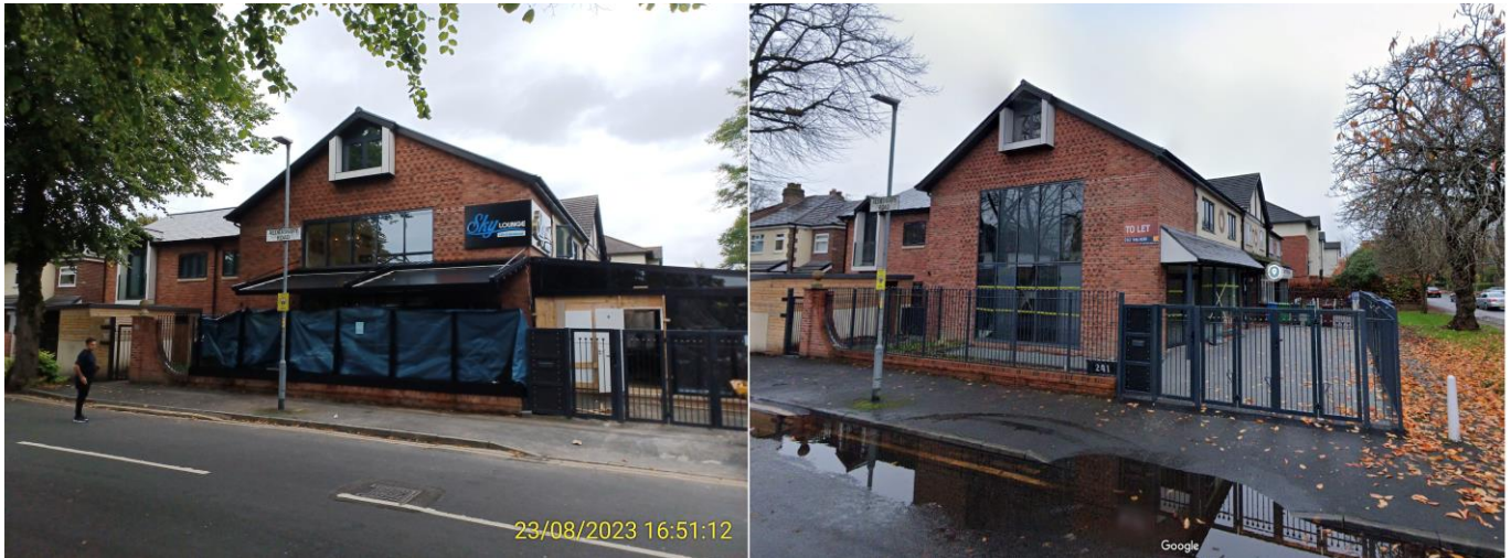
Photograph 4 and Image 3 Comparison of before and after side awning photograph as dated, Source: Case Officer Site Photograph and Google Streetview prior to the installation of the front extension and retractable side awning dated Nov 22. Source: www. https://www.google.com/maps/@53.4269436,-2.2599199,3a,47.5y,255.59h,92.2t/data=!3m6!1e1!3m4!1sCAgNw3xKo52zMkrb_A91Mq!2e0!7i16384!8i8192?entry=ttu
