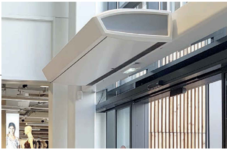
TYPICAL INSTALLATION OF PROPOSED OVERDOOR HEATER
