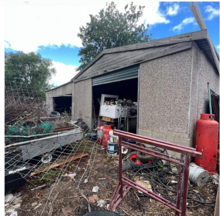
Photo No.6: Facing NW from the SE corner of the garage
