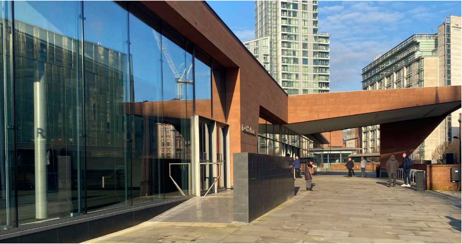
Close up view of existing step and ramp arrangement leading to a fire escape, directly adjacent to the main entrance to the venue.
