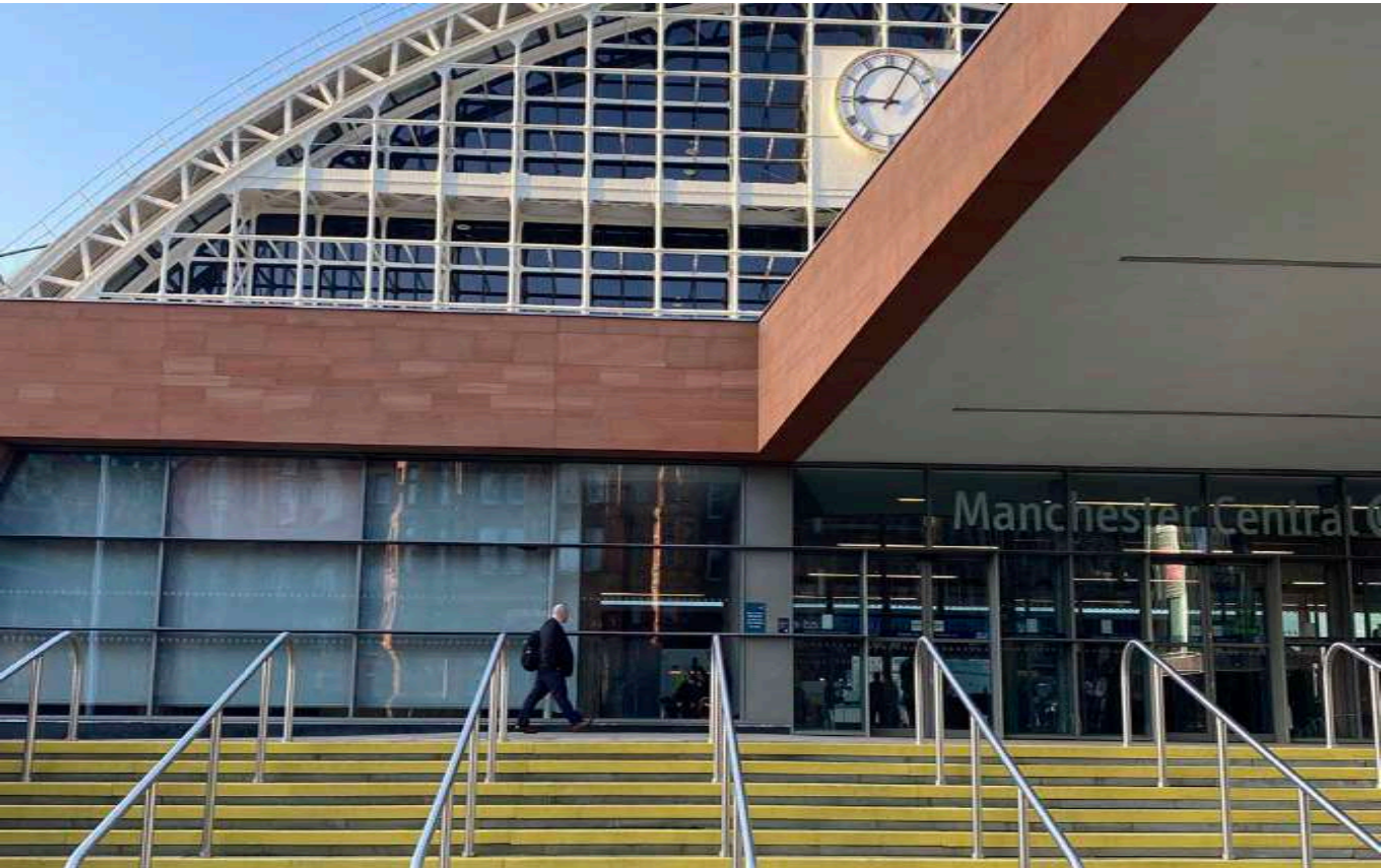
Close up of main entrance to venue with Cobden Rooms site to the left.
