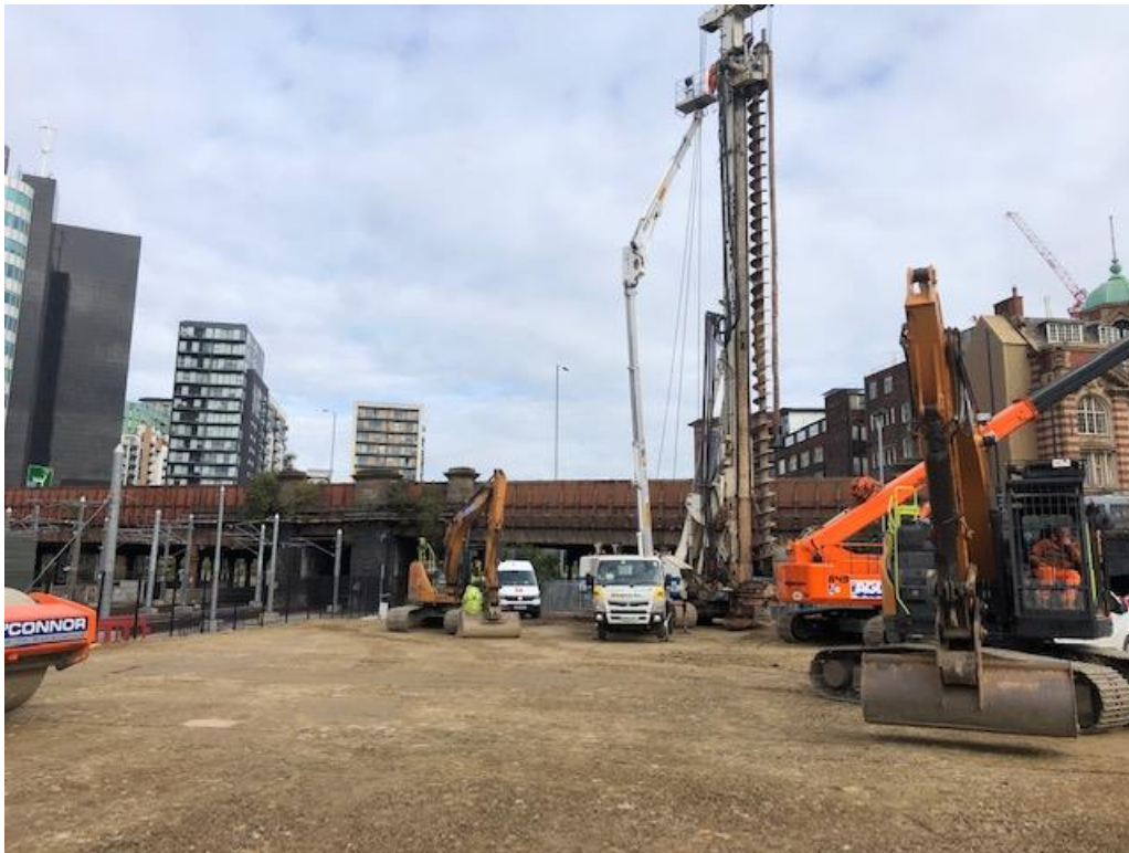
PLATE 7 WORKING PLATFORM CONSTRUCTED WITH MPORTED 6F2
