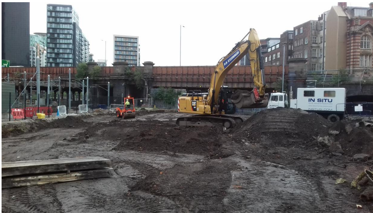
PLATE 4 EXCAVATION, BREAKING OUT AND PROCESSING
