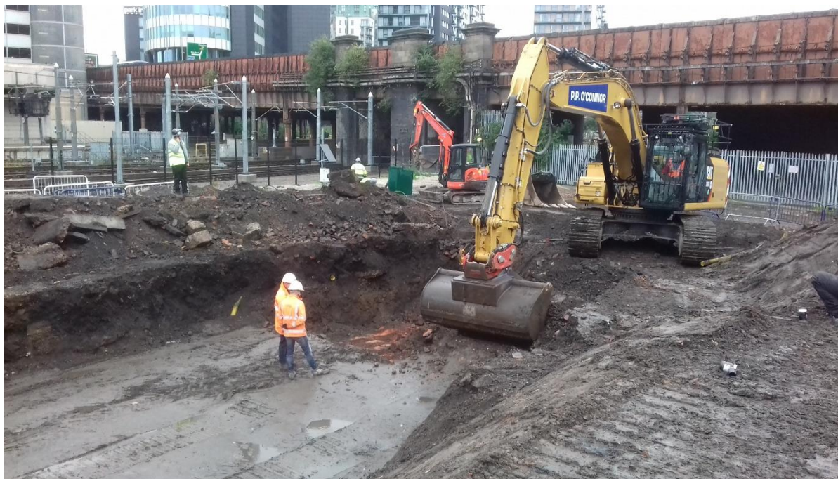
PLATE 2 EXCAVATION, BREAKING OUT AND PROCESSING
