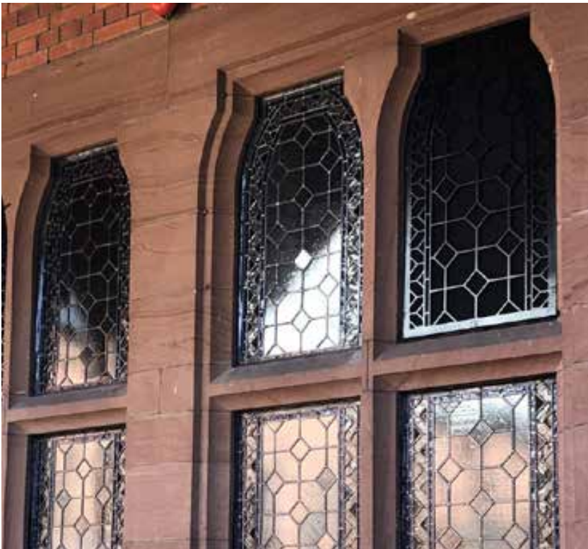
Top left and right - Photograph of inside and outside of existing vent/ leaded light. Bottom - Precedent photograph of decorative grille/ vent replicating the pattern of an adjacent leaded light.
