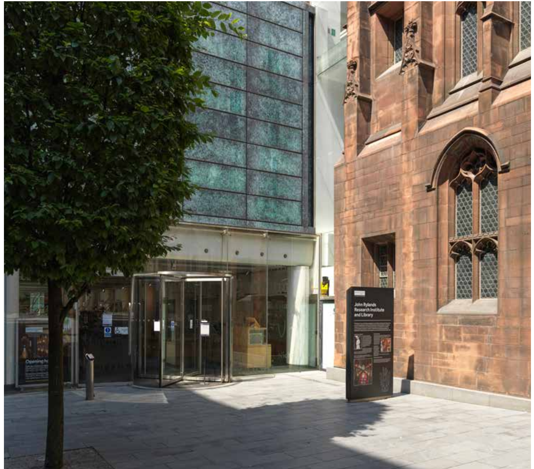
Photograph of existing modern entrance and revolving door (part of the to 2007 extension).
