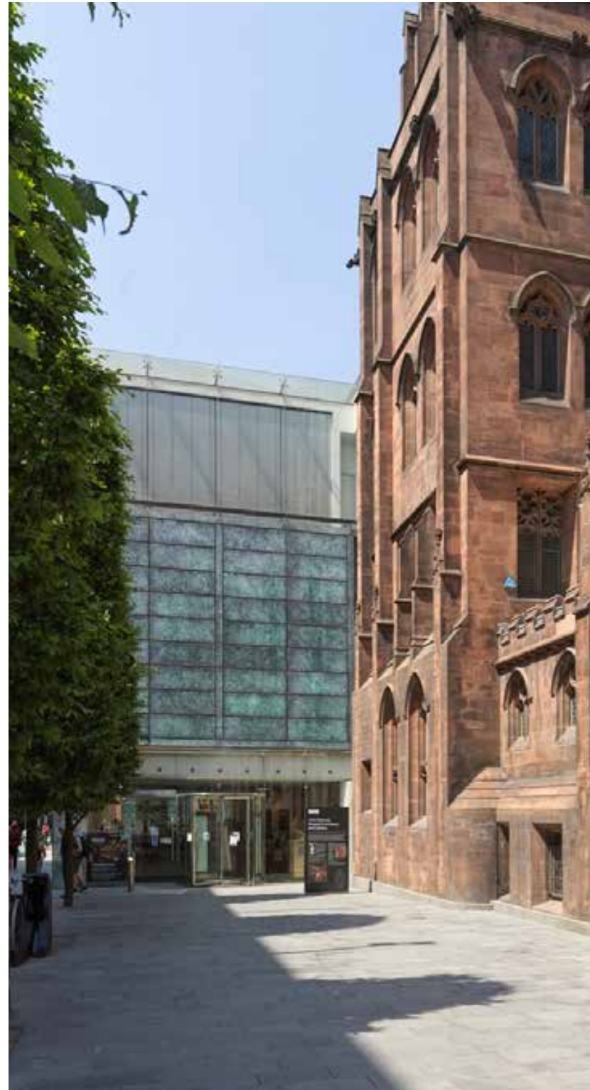
Photograph of existing modern entrance (part of the to 2007 extension).
