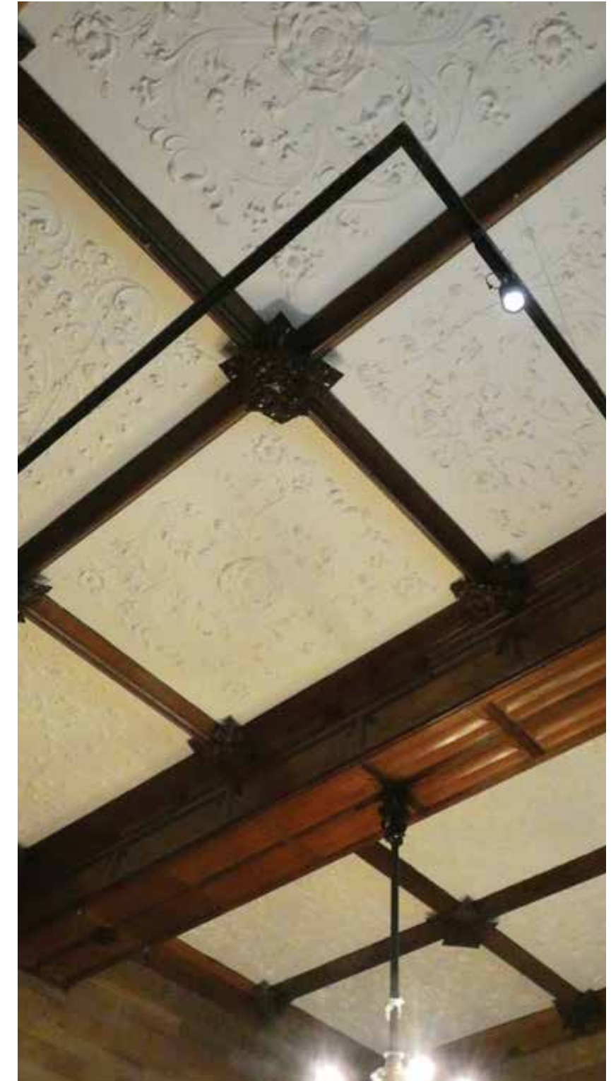
Photograph of existing room, including modern track lighting.
