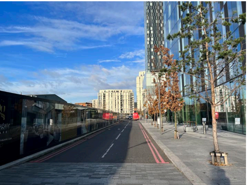
View looking north along Owen Street with timber hoarding lines around the Phase 3 site
