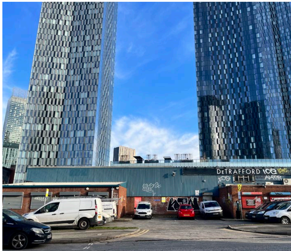
View of Crown Street Phase 3 eastern parcel from Great Jackson Street (Deansgate Square in the background). Site photo taken prior to clearance.
