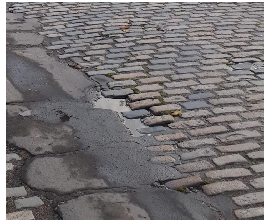
Existing materials and condition of Silvercroft Street
