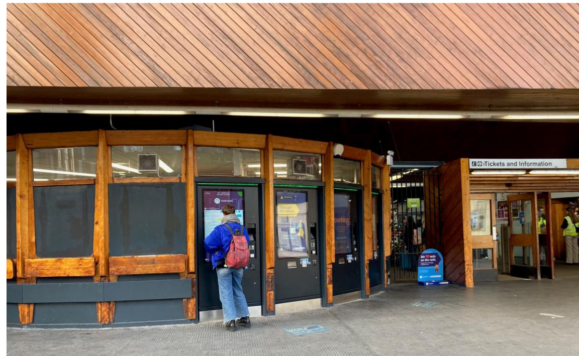
Existing roof line around area where proposed CIS screens are to be located
