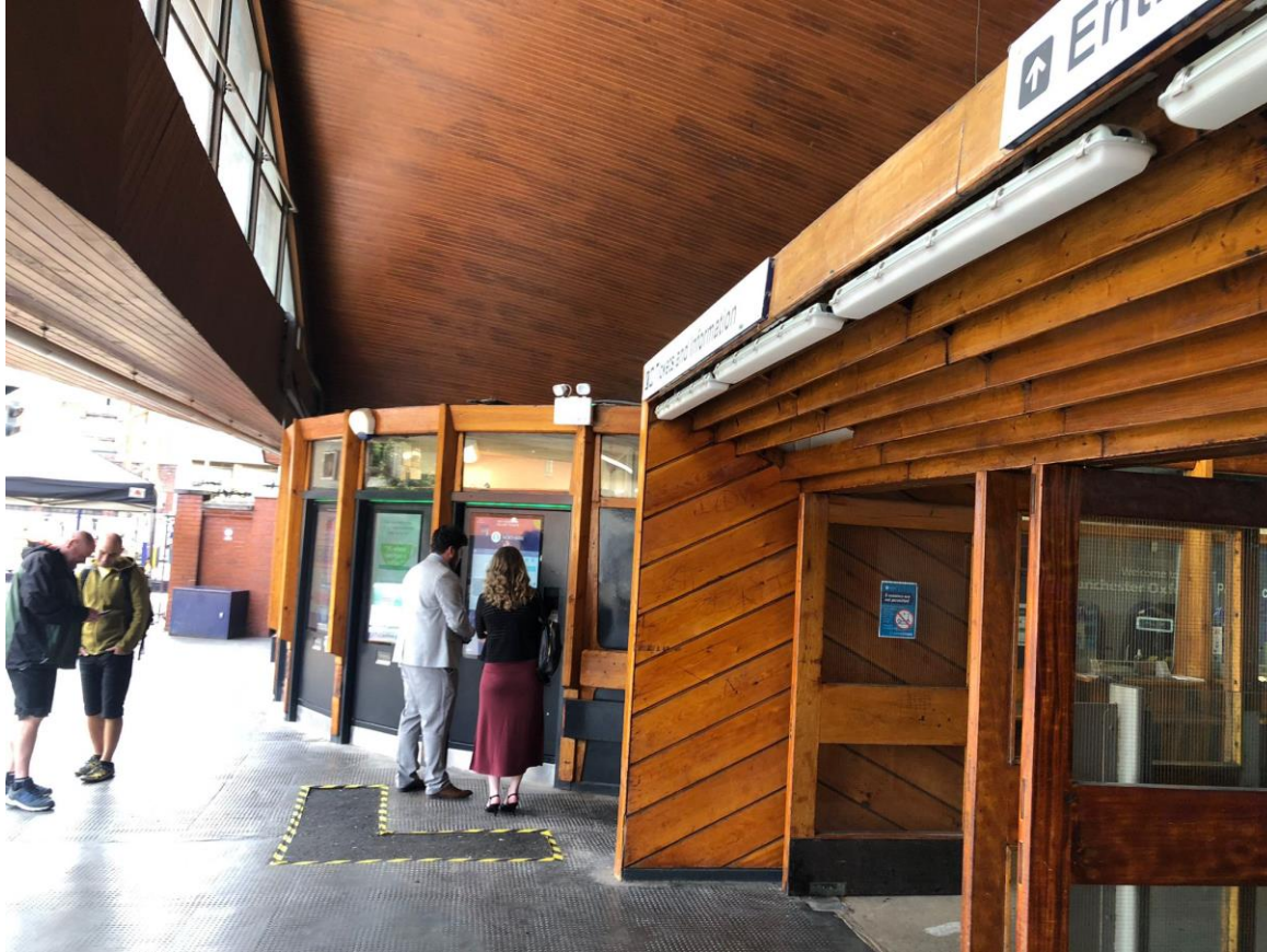
Existing roof line around area where proposed CIS screens are to be located
