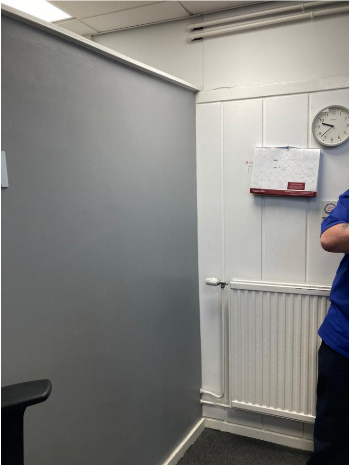
Existing ticket office showing far end of 'hockey stick' ¾ height wall.
