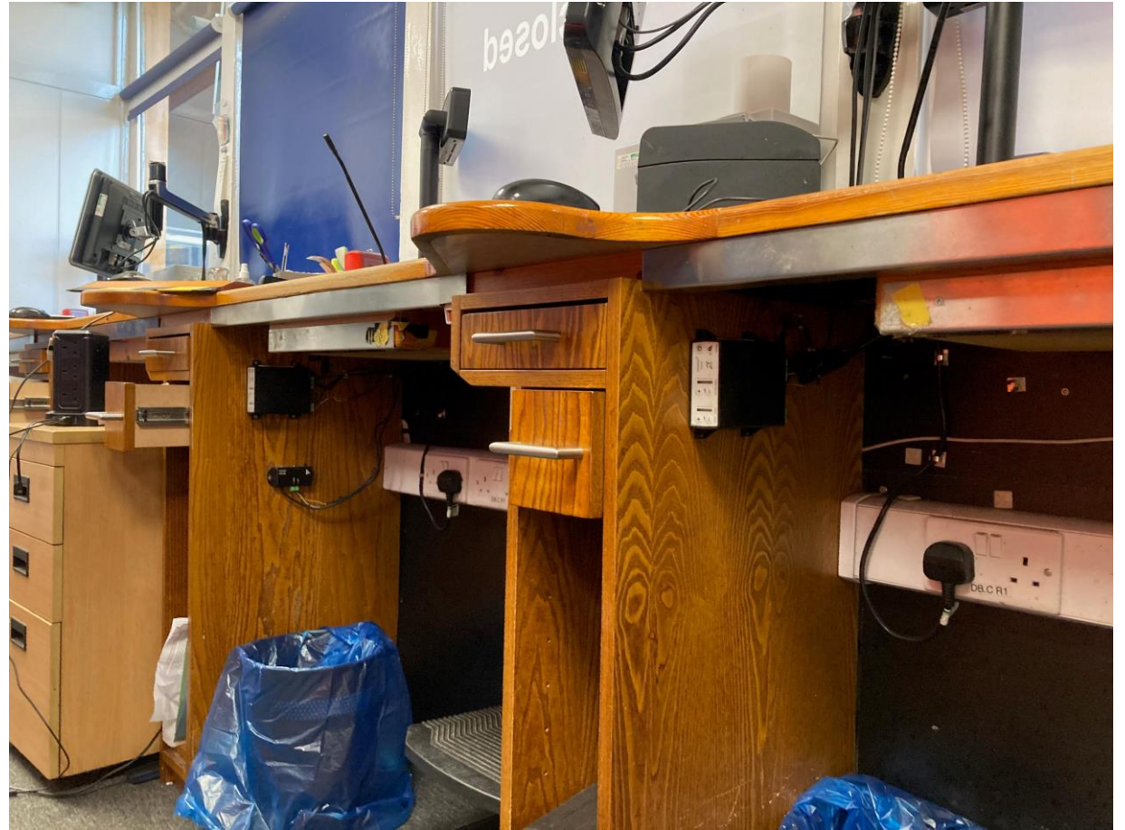
Existing ticket office, showing underside of existing ticket desk.
