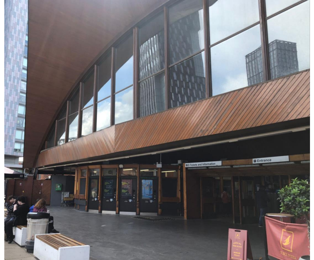
Existing Station frontage, from pedestrian entrance.
