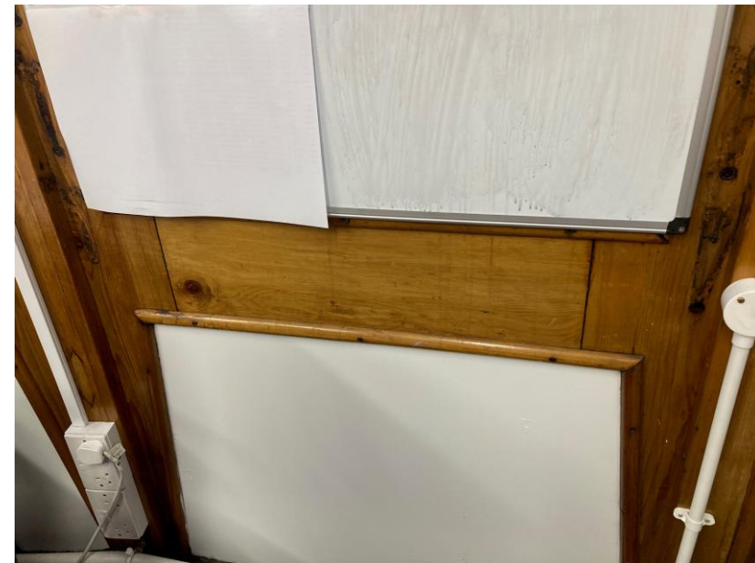
Existing internal face of the lozenge in the existing station managers office, to become the proposed ticket office. Image showing the waist height area internally.
