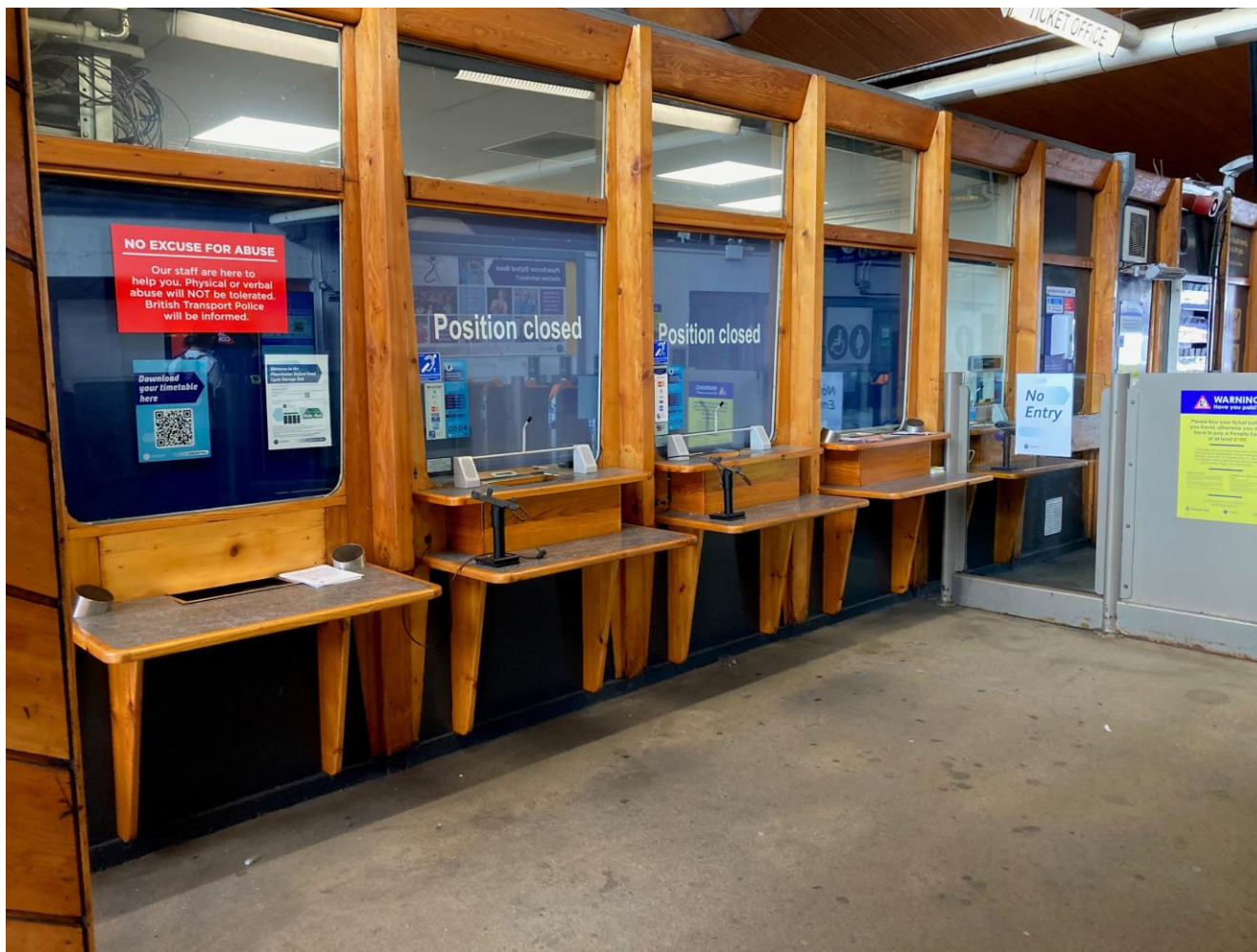
Existing 5no. ticket desks, with far desk located behind glazed screen on paid side.
