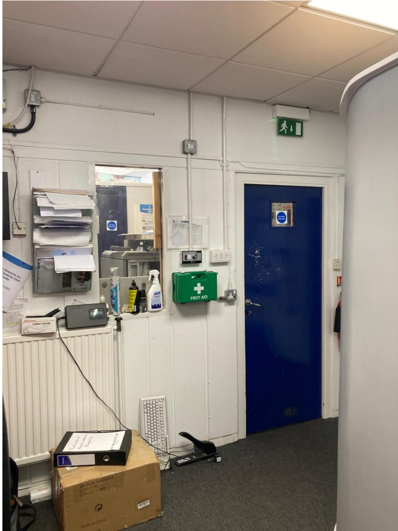
Existing ticket office showing existing entrance door. Proposed wall to sit next to door.
