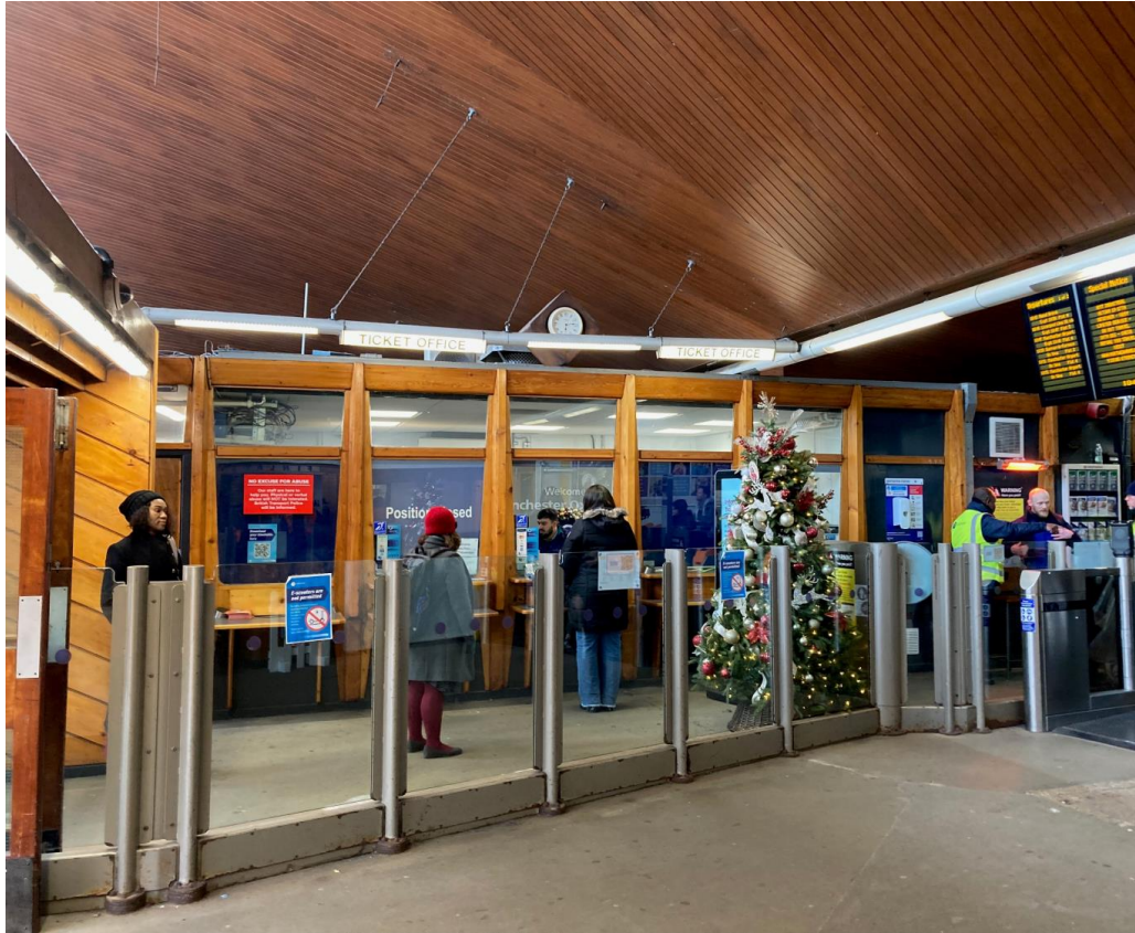
Glazed separation screens in front of the existing ticket desks.
