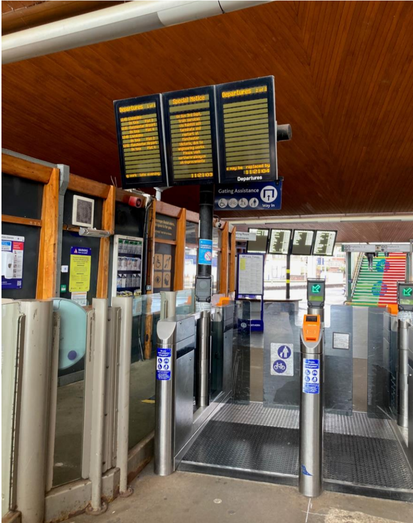
Existing 3no. CIS screens mounted on a 'T' support column.
