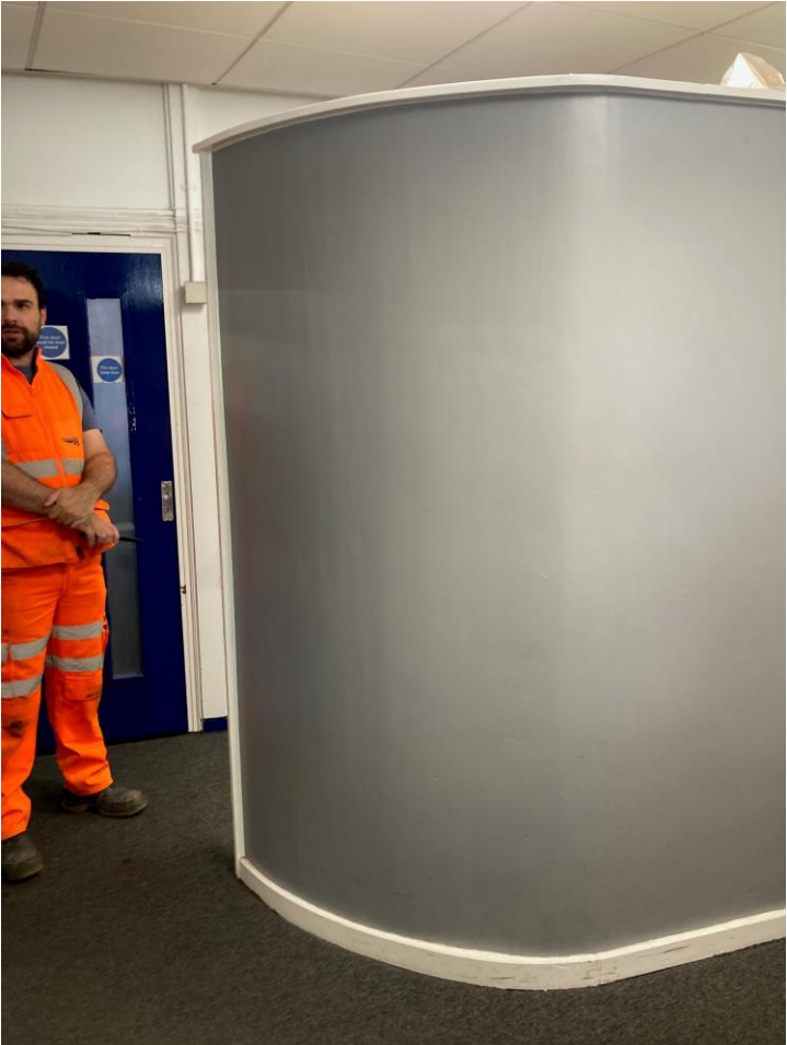
Existing ticket office showing end of 'hockey stick' ¾ height wall from ticket counter side.
