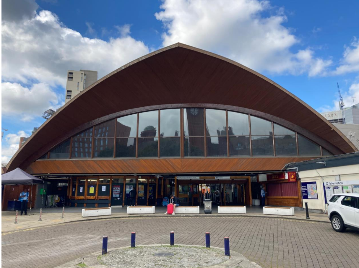
Existing Station frontage, from central traffic island.
