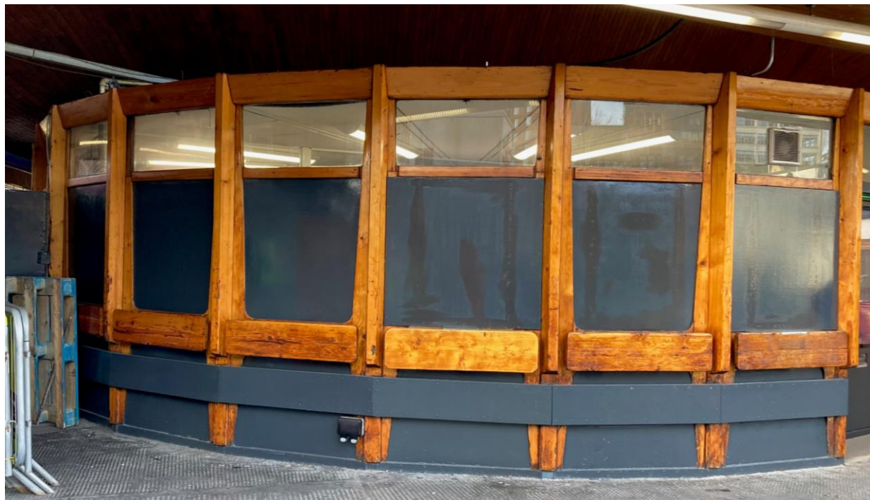
Existing Station frontage at the site of the 2no. proposed ticket desks.
