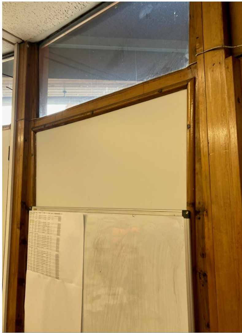
Existing internal face of the lozenge in the existing station managers office, to become the proposed ticket office.
