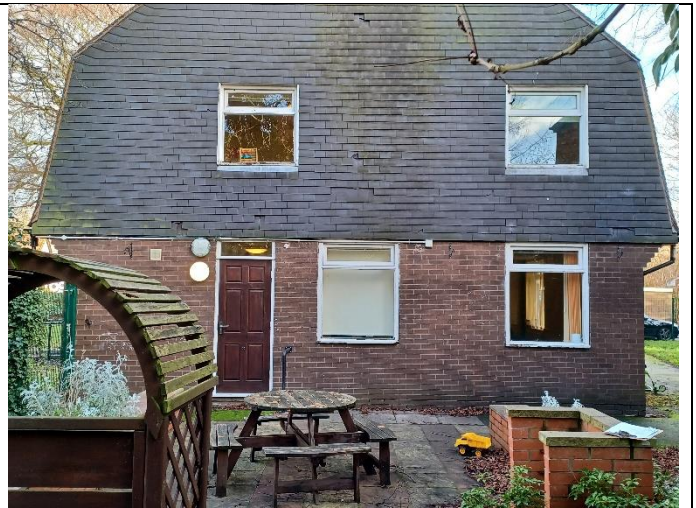
A new door opening & ramp to this elevation.
