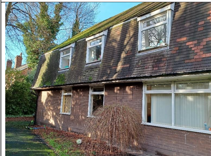
A new door opening & ramp to this elevation also.
