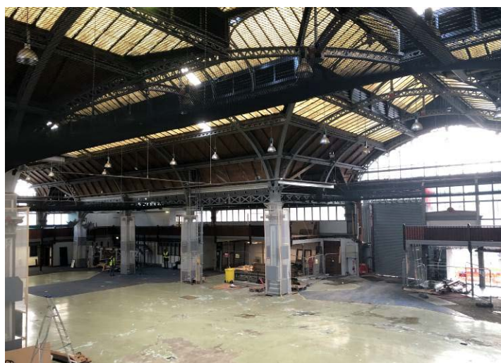
Figure 89: Looking south-east across the building towards the southern elevation.
