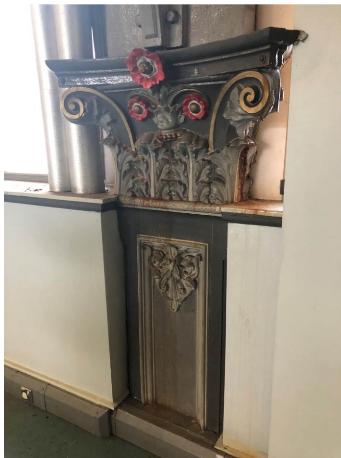
Figure 112: An example of one of the original decorative cast iron external columns, showing a representation of a Lancashire rose to the capital.
