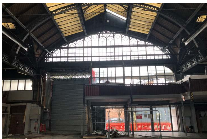
Figure 88: The central section of the south elevation.
