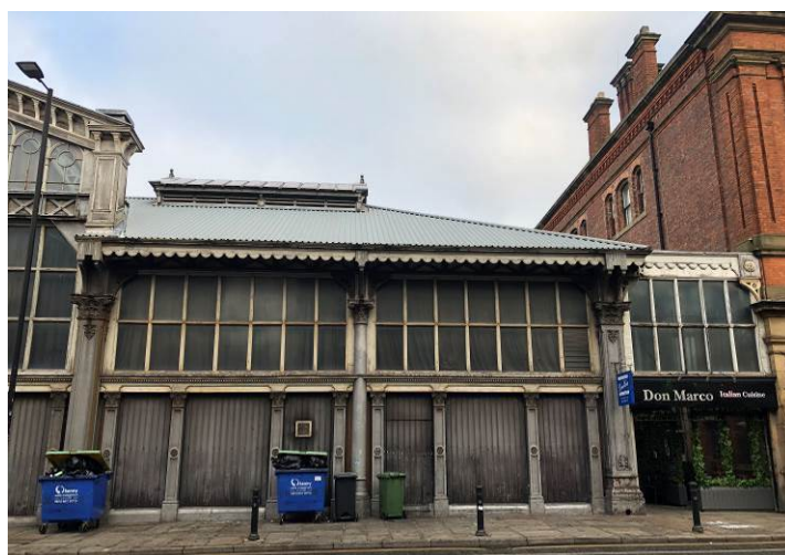
Figure 44: The eastern section of the south elevation, showing the matching link that connects the market building with the former library building (right) across a former market alley.
