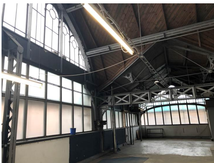
Figure 111: Looking north along the western mezzanine.
