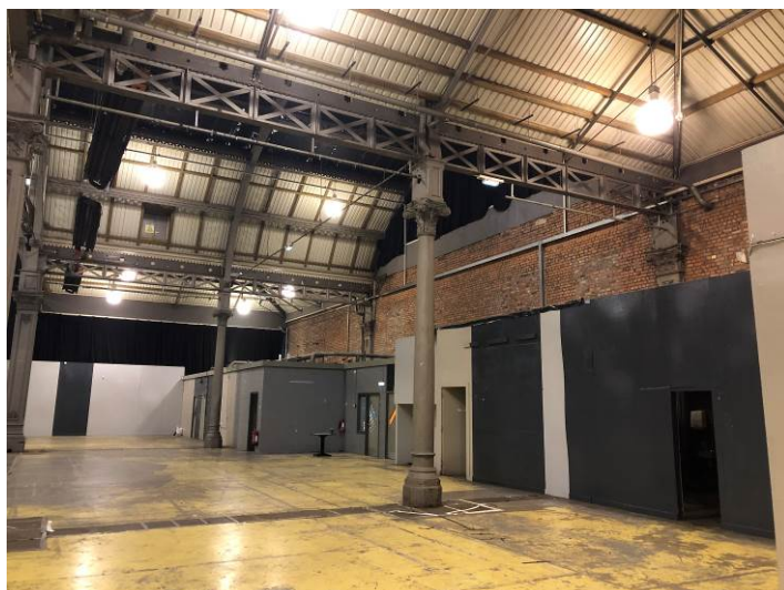
Figure 67: Looking east towards the east elevation showing the two modern (c1980s) enclosures forming toilets, kitchen and office etc. This part of the market formed the 1894 fruit auction room (to roof level), with ground floor shops below.
