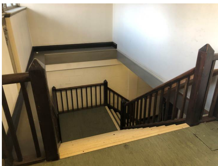
Figure 113: An example of one of the four 1980s mezzanine staircases located to each corner of the building.
