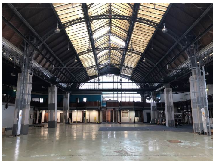
Figure 98: Looking east across the building towards the east elevation.
