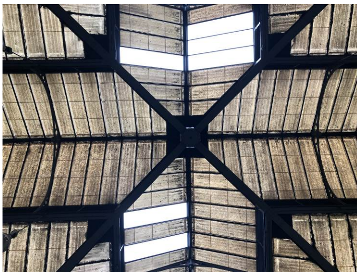
Figure 104: An example of the modern 1980s fibreglass panels (discoloured) and more recent clear coverings to the centre of the roof.
