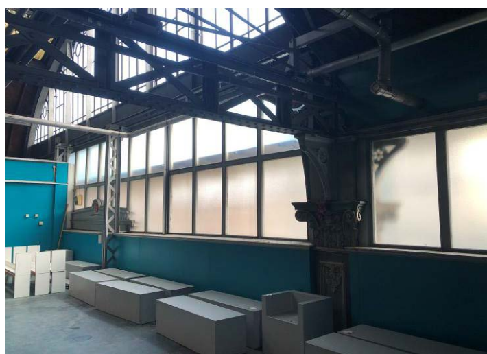
Figure 108: The eastern side of the southern mezzanine.
