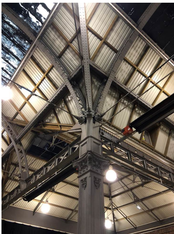
Figure 75: An example of the decorative original central columns, which feature decorated composite capitals.
