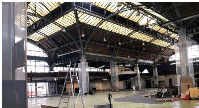
Figure 87: Looking south-west across the building towards the southern elevation.
