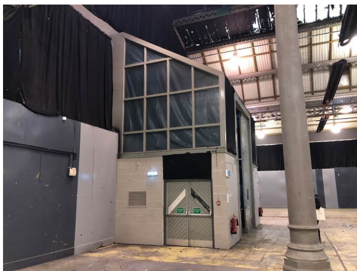
Figure 66: Looking west along the southern elevation of the building, showing one of the two modern (c1980s) entrance enclosures.
