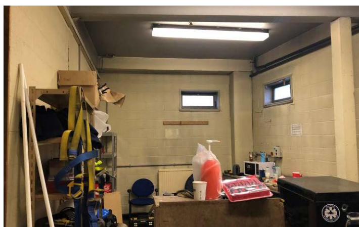
Figure 97: A 1980s room located to the south-west corner of the ground floor.
