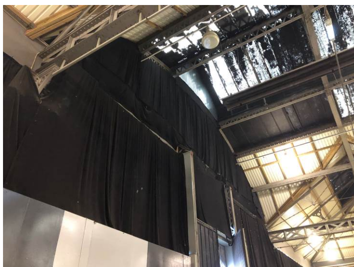
Figure 63: Looking up to the modern curtains that now conceal the original Venetian glazed gable end onto Tonman Street.
