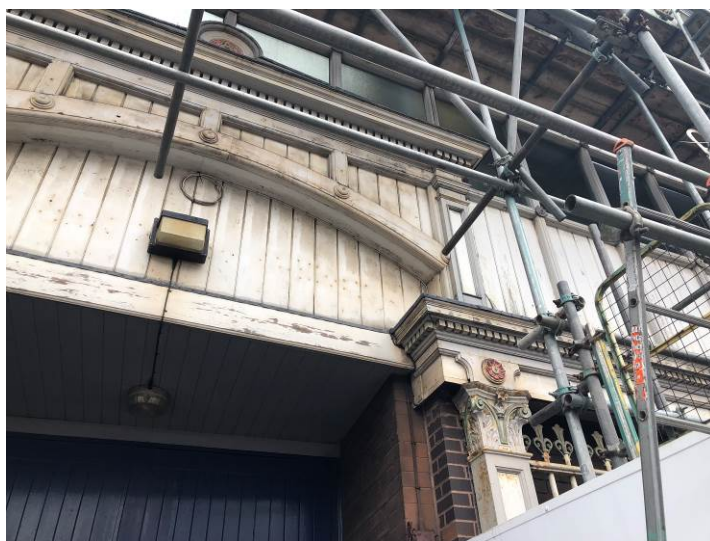
Figure 82: The lower parts of the west elevation.
