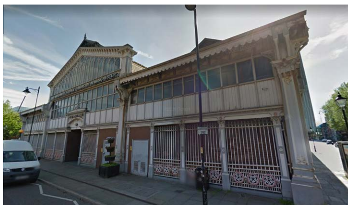
Figure 81: The southern elevation as seen from Lower Byrom Street. (2018)
