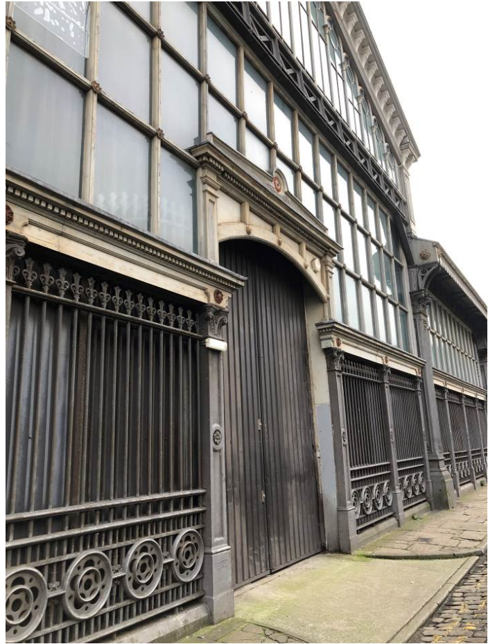
Figure 49: The central entrance to the west elevation on Barton Street, showing the only examples of surviving original cast iron railings to the bottom part (left and right). Although the central gates are modern, the original cast iron railed gates survive behind the corrugated metal within the side elevations.
