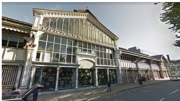
Figure 77: The central, raised portion of the southern elevation, showing original cast iron Venetian windows to gable and modern glazed openings to lower portions in the place of removed original cast iron railings. (2018)
