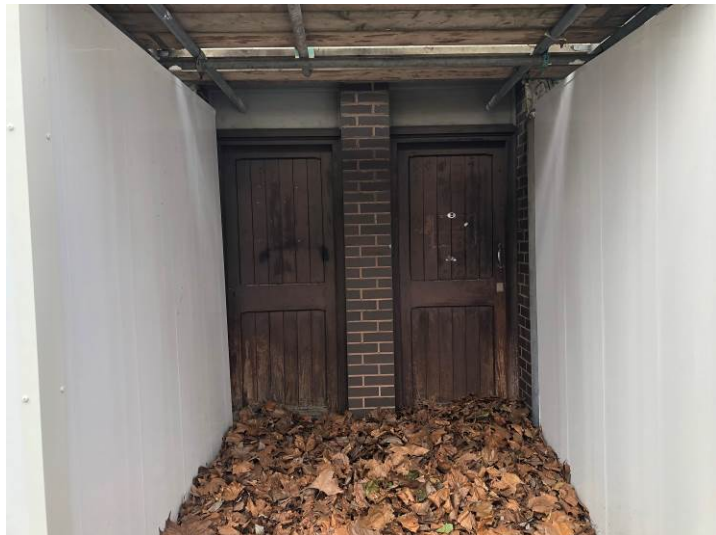
Figure 86: Examples of 1980-3 doors to the east elevation.
