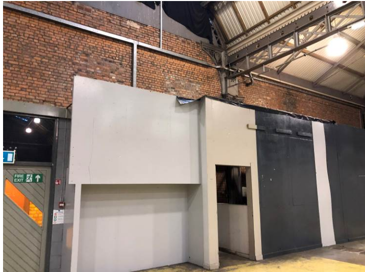
Figure 68: The east elevation showing the modern (c1980s) enclosures.
