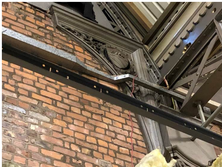
Figure 69: A detail of the upper part of the east elevation, showing the c1880s brickwork encapsulating the 1870s cast iron framework. Note the decorative foliage and Manchester coat of arms to the bracket, which depicts three lines representing the three rivers which run through Manchester city centre: the Irwell, the Irk and the Medlock, with a ship in full sail above.
