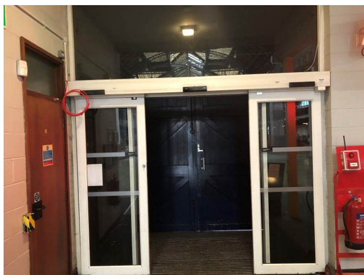
Figure 96: The modern entrance vestibule to the west elevation.
