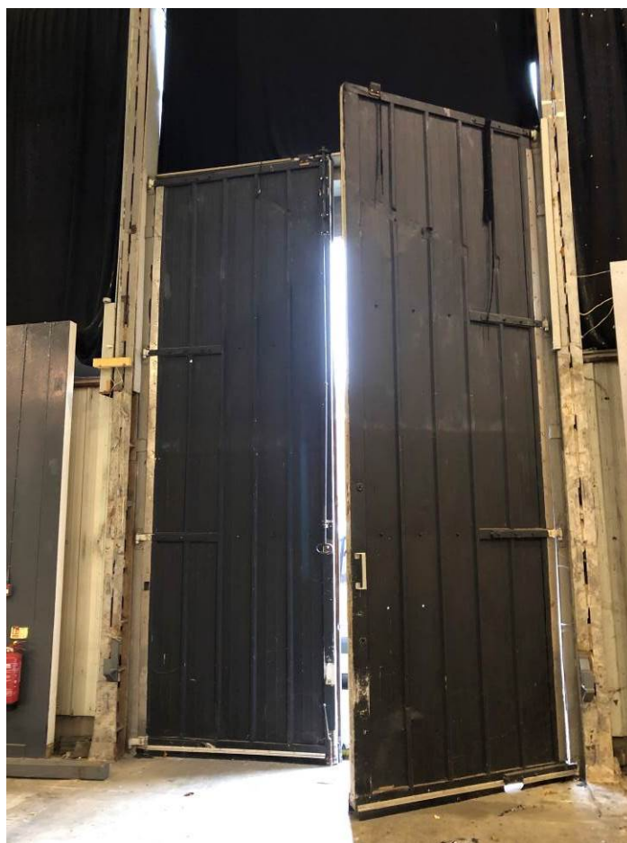
Figure 62: The modern corrugated metal gates onto Tonman Street.
