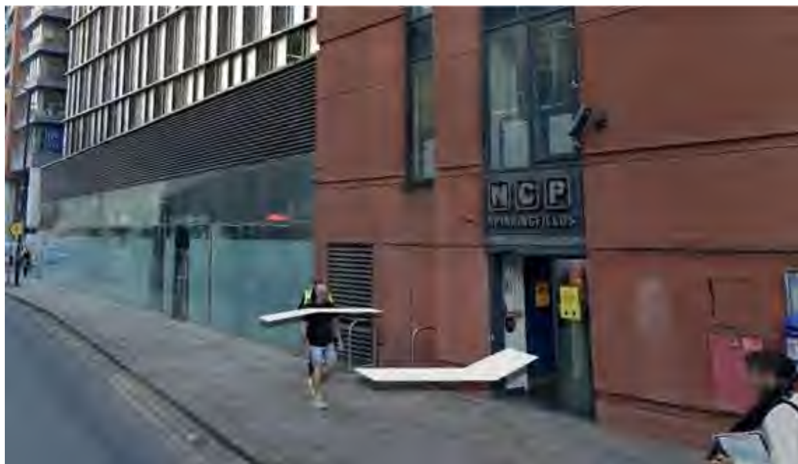
Figure F.2: The Off-Site Entrance(s) at Point 29
