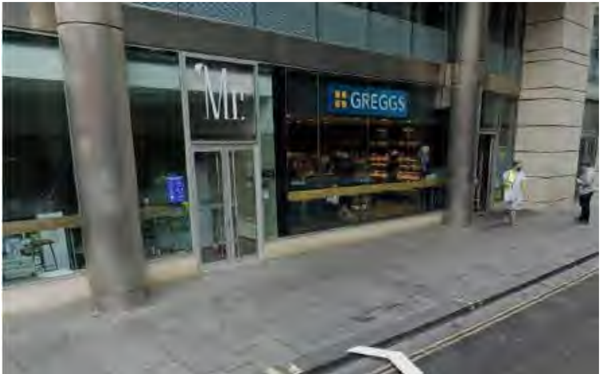
Figure F.3: The Off-Site Entrance(s) at Point 31
