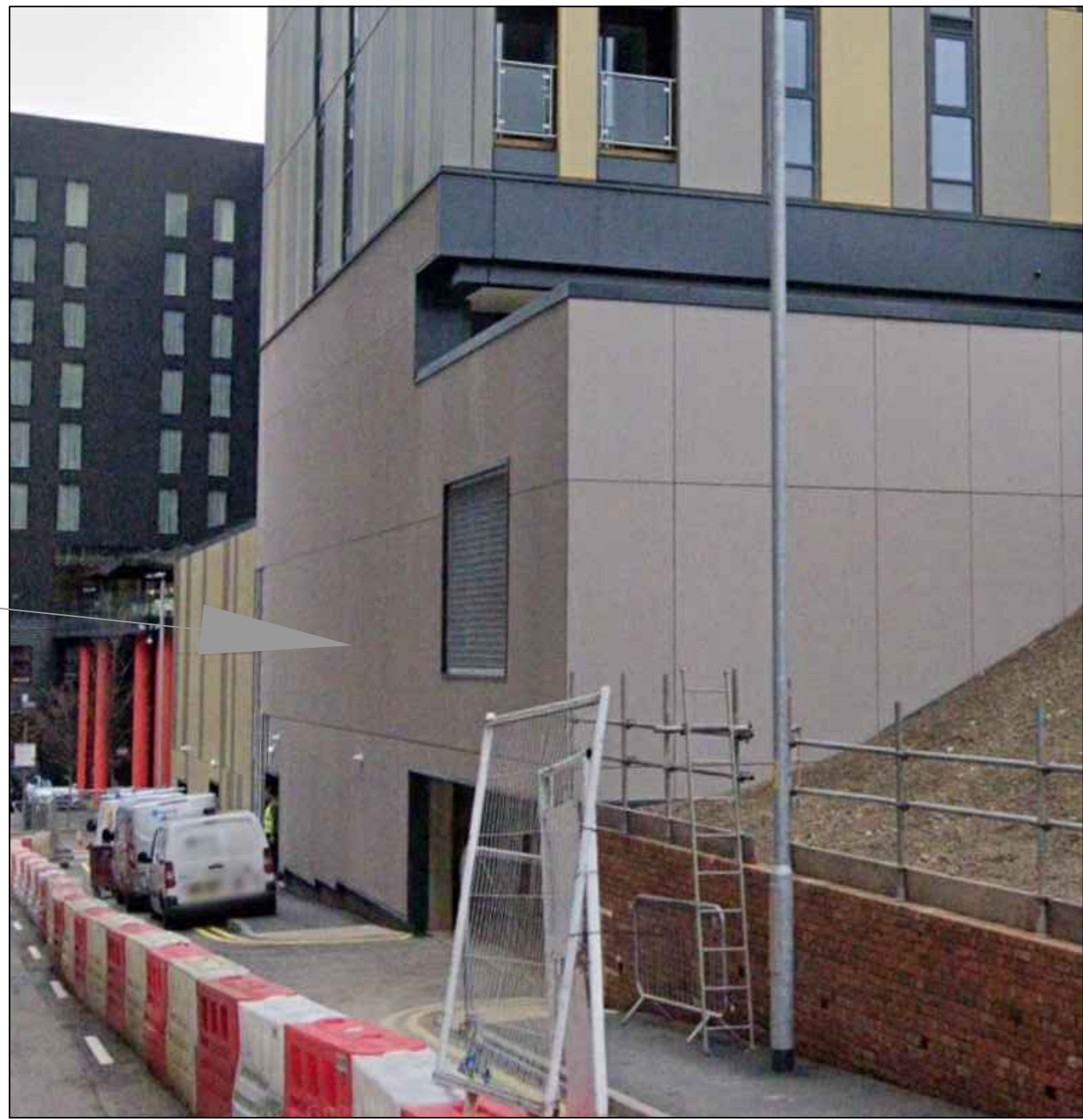
APPEARENCE OF CLADDING
