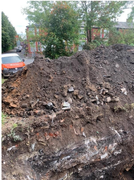
PLATE 4 EXCAVATION FOR CULVERT TRENCH (EASTERN SECTOR)
