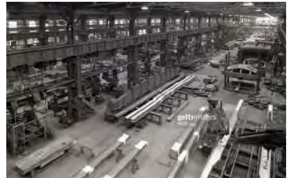
View of the press bay and middle bay of the boiler shop, 1959, Beyer Peacock Works.
