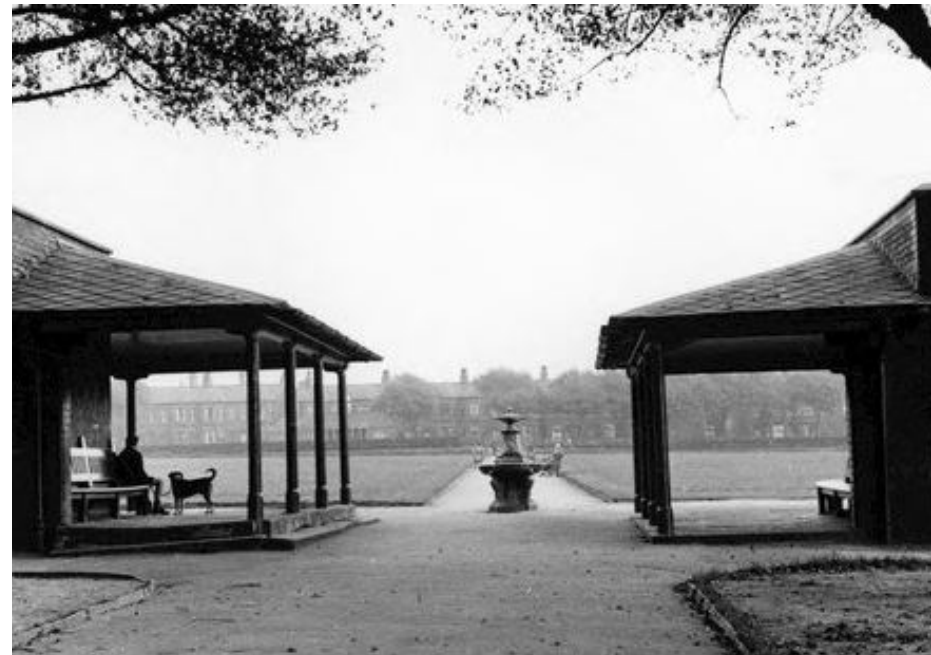
Delamere Park Shelter c.1955
