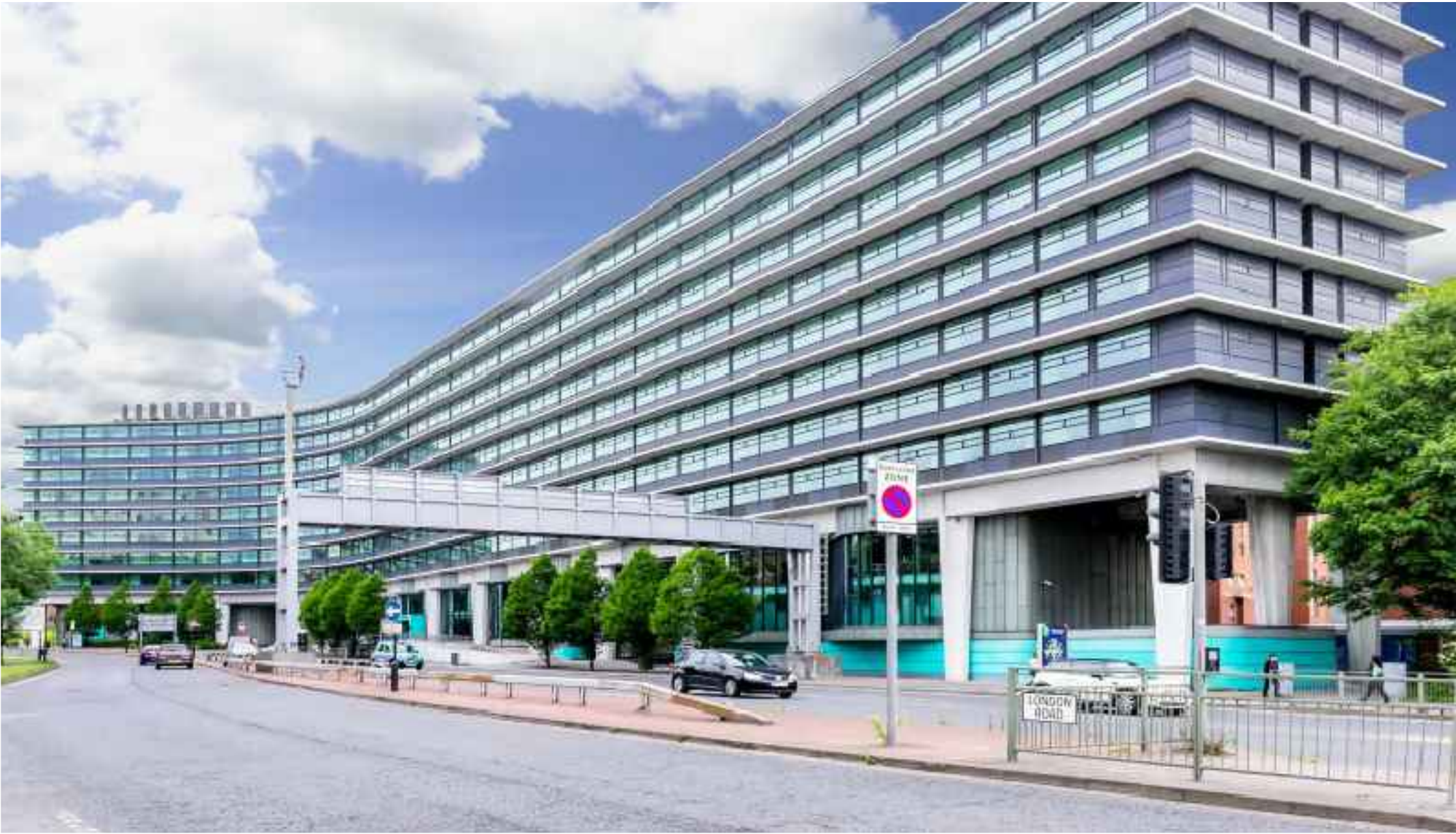
VIEW OF FRONT ELEVATION SHOWING BLANK END ELEVATION FACING AWAY FROM PICCADILLY STATION
