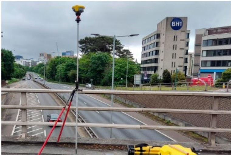
7: Field survey being carried out, GNSS receiver
