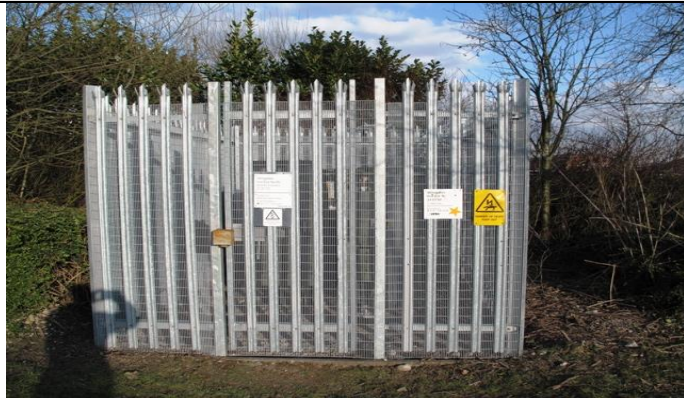
Example Security Upgrade Works and Earthing Installations
