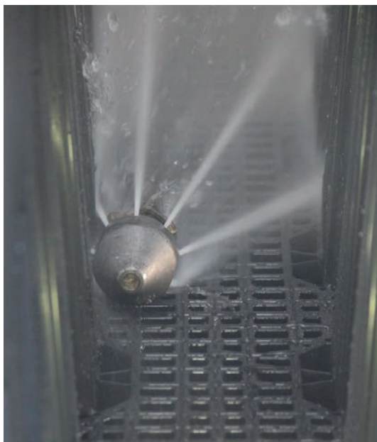
Figure 12 - Jetting nozzle flushing the system
