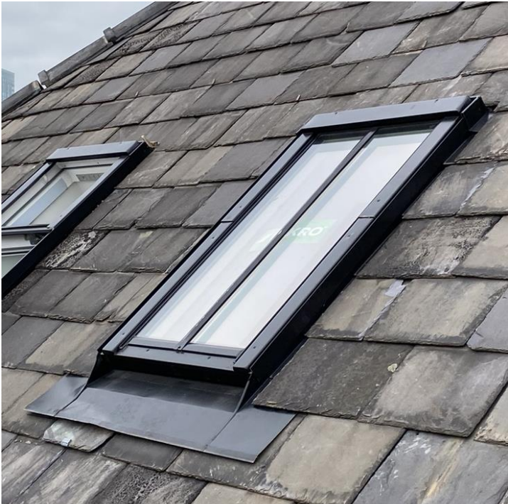
Fakro aluminium clad PVC glazed rooflight installed
