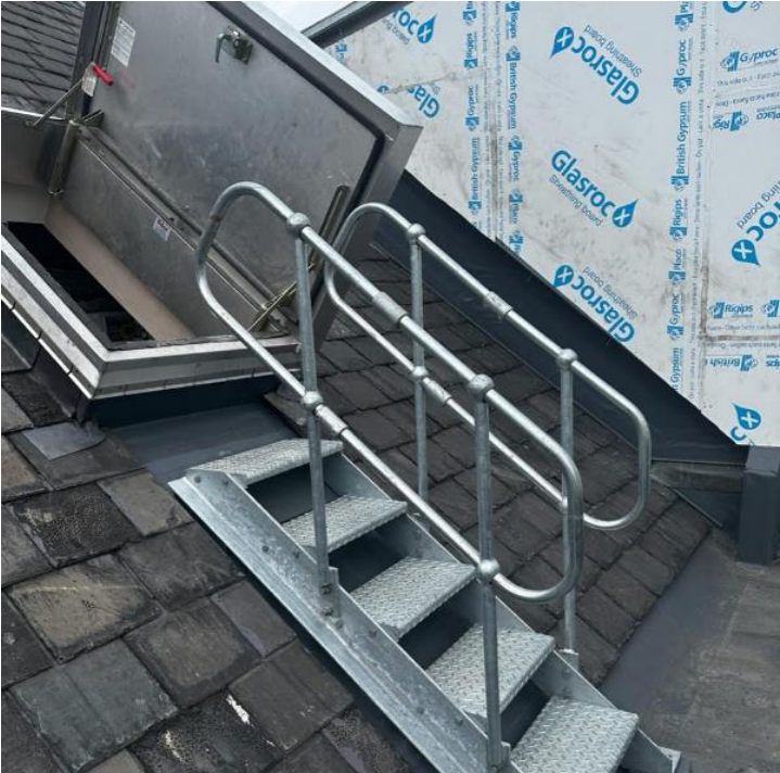
Bilco roof access hatch installed pitched roof with bespoke ladder
