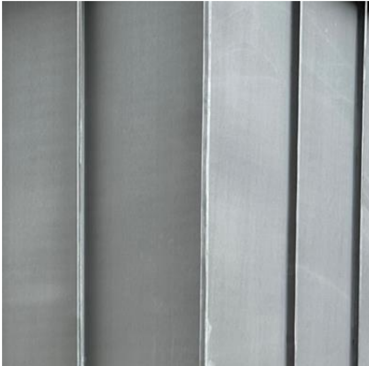
VM Zinc standing seam cladding to lightwell lift/stair enclosure
