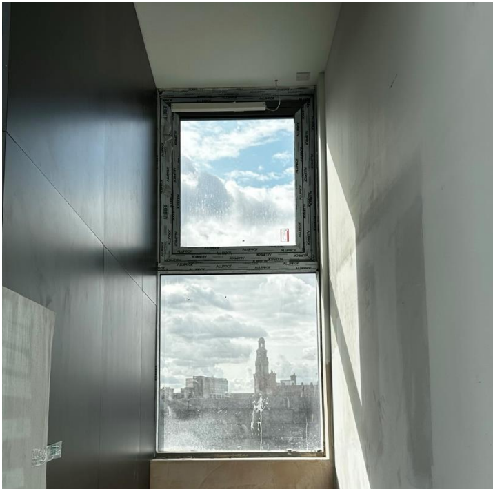
Aluminium framed glazed automatic opening vent installed
