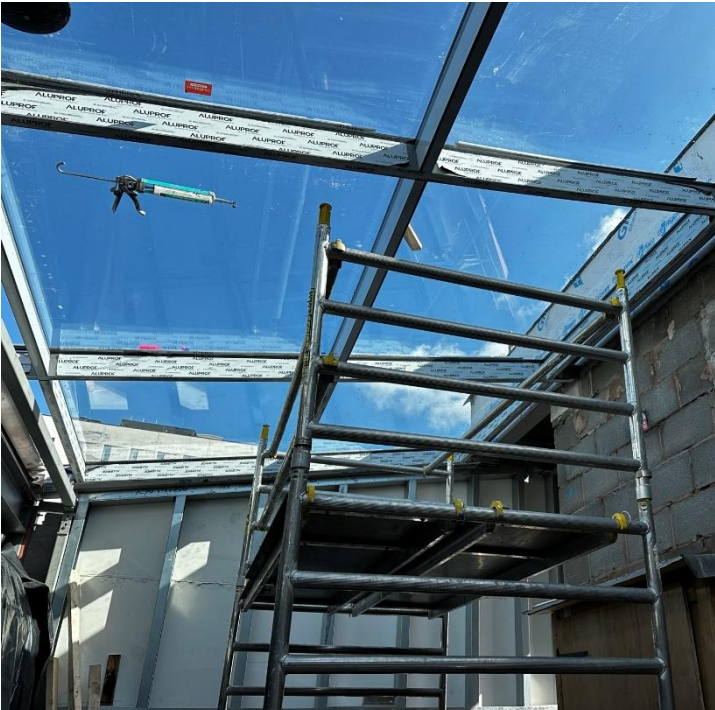
Aluminium framed glazed rooflight to lightwell installed
