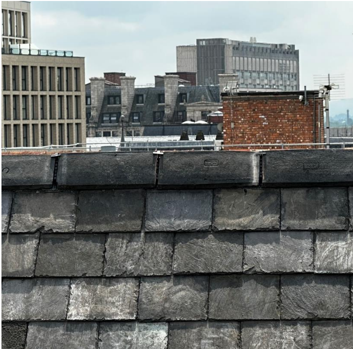
Marley ventilated ridge system with existing tiles installed
