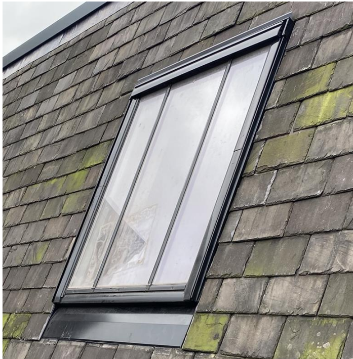
Velux aluminium clad timber framed glazed rooflight installed
