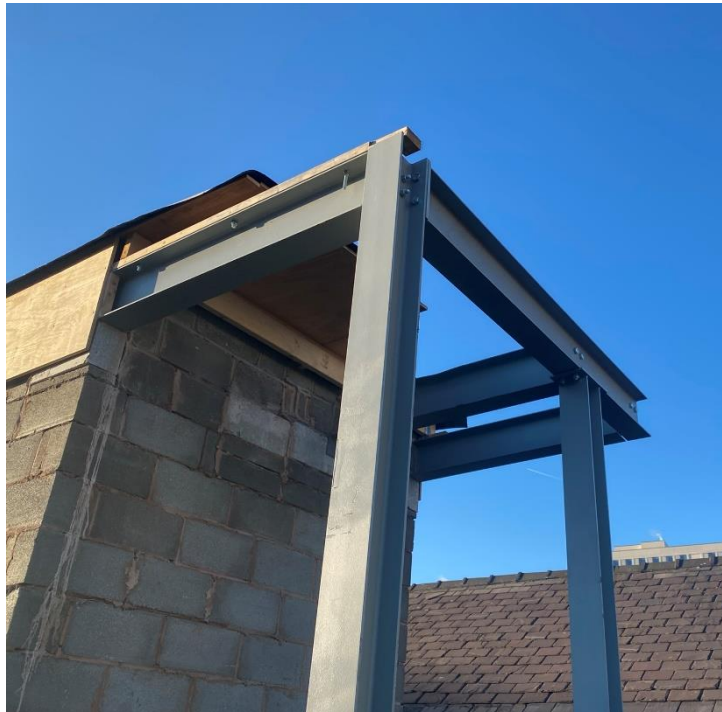
Blockwork lift shaft with steel frame to form lightwell enclosure
