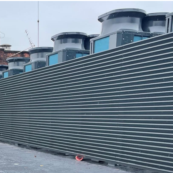
Caice aluminium louvred plant screen installed
