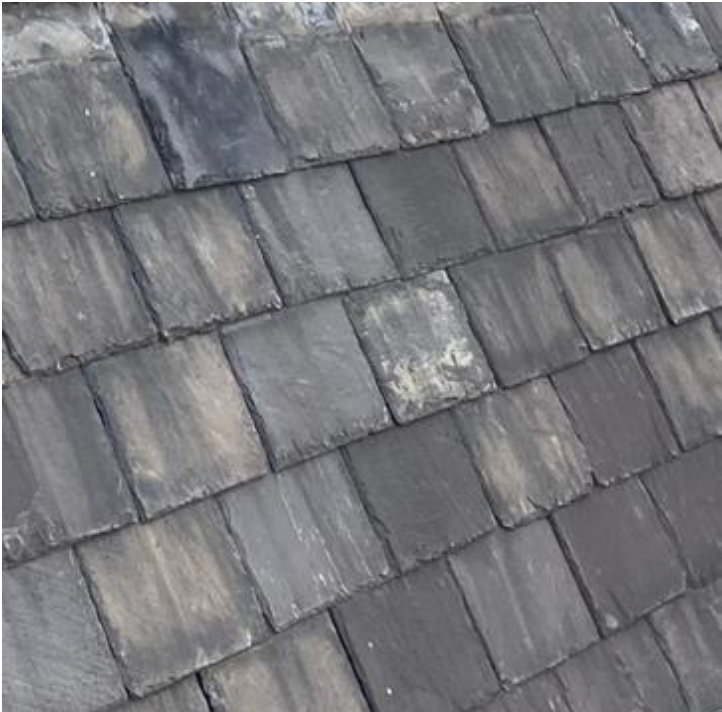
Original pitched roof slates re-purposed to clad new mansard roof
