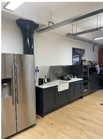
Figure 12: Second Floor, kitchenette. Original columns ( high significance ). Modern ductwork and modern kitchen fixtures.
