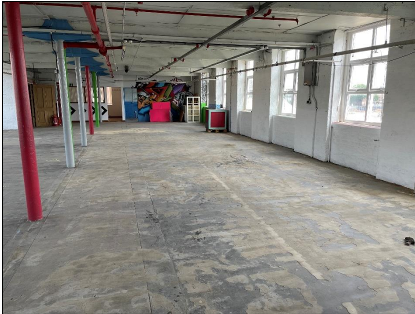
Photograph 4 showing one of the open floors
