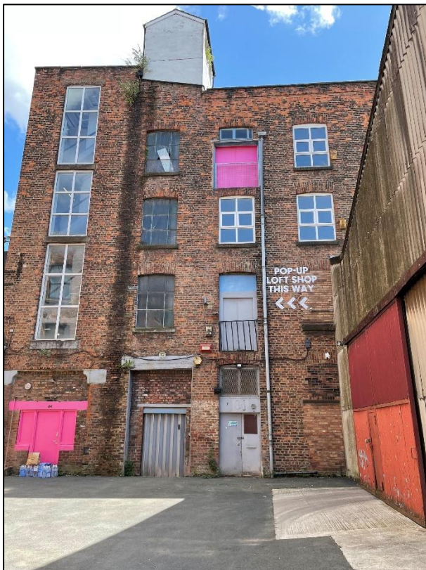
Photograph 2 showing the northern elevation (the lift gear shed can be seen)
