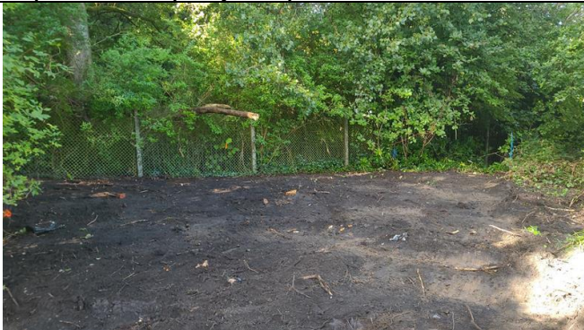
100mm scrape of Japanese Knotweed within RPA completed
