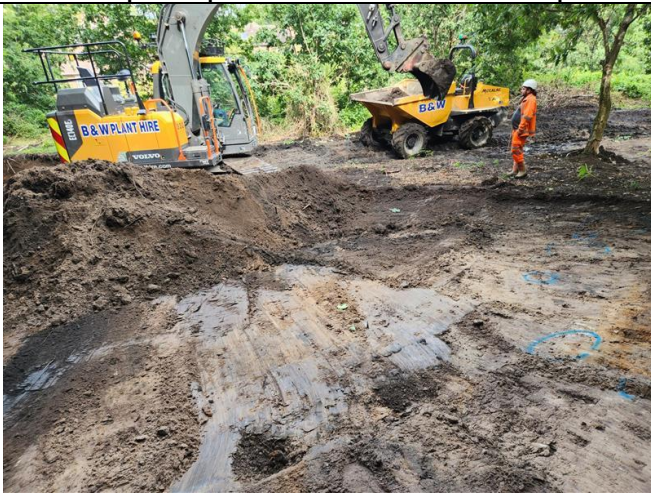
100mm scrape of Japanese Knotweed within RPA completed
