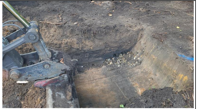
Excavation of Japanese Knotweed impacted soils
