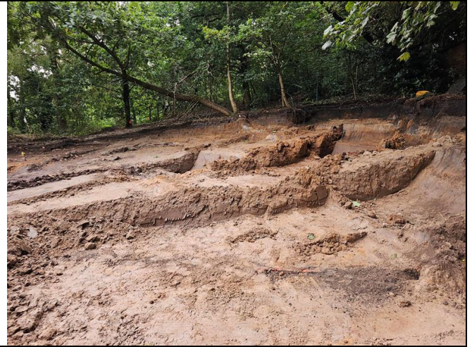
Excavation of JK completed
