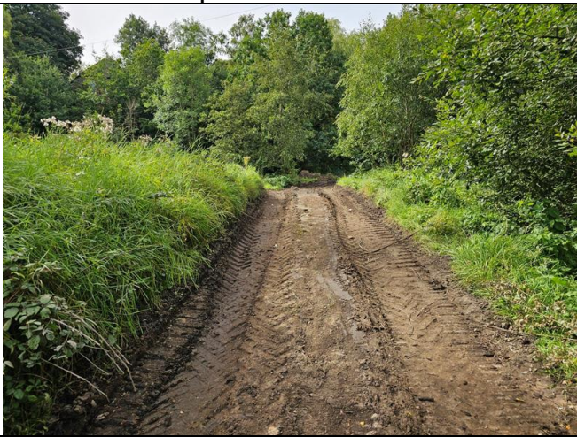
Scrape of haul road completed.
