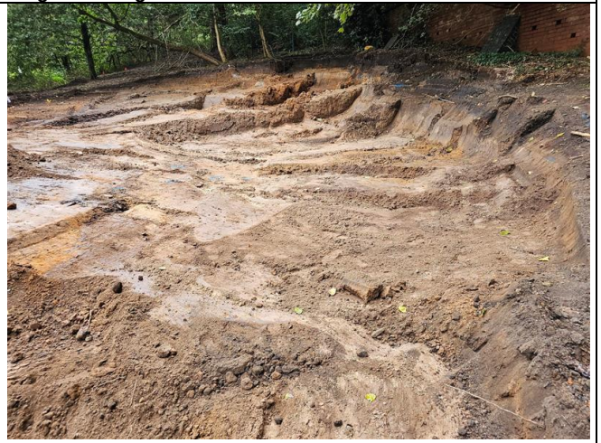
Wagon loading commenced
