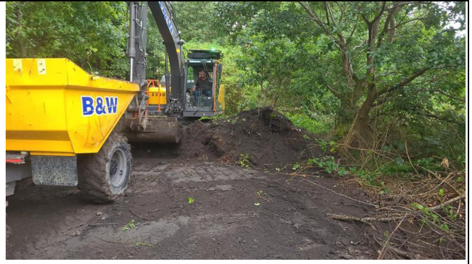
Excavation of intrusive survey stockpiles
