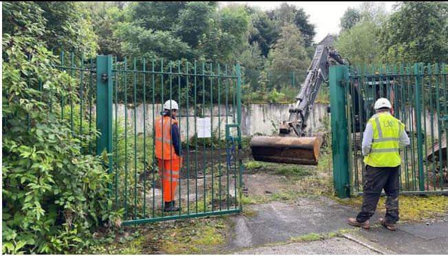
Preparation of temporary stockpile area
