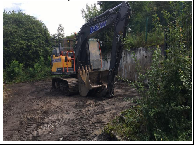
Scrape of temporary stockpile area completed
