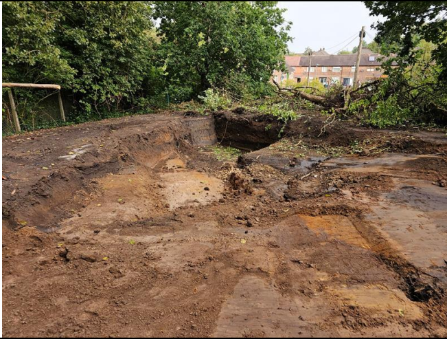
Excavation of JK completed
