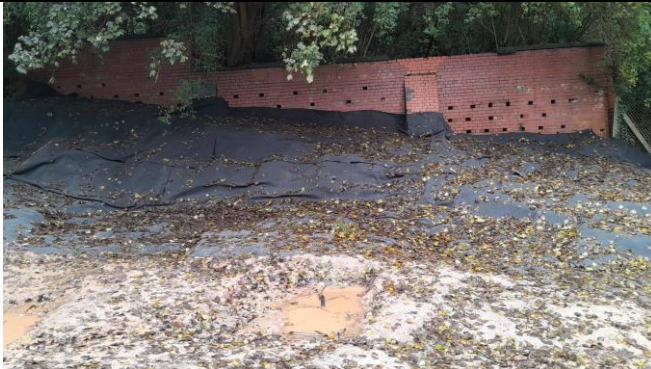
Installation of geo-textile root barrier completed
