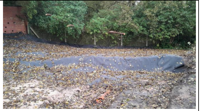
Installation of geo-textile root barrier completed
