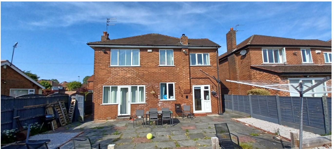
Figure 3. Rear of property.
