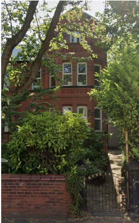
Existing Pedestrian Entrance to the site
