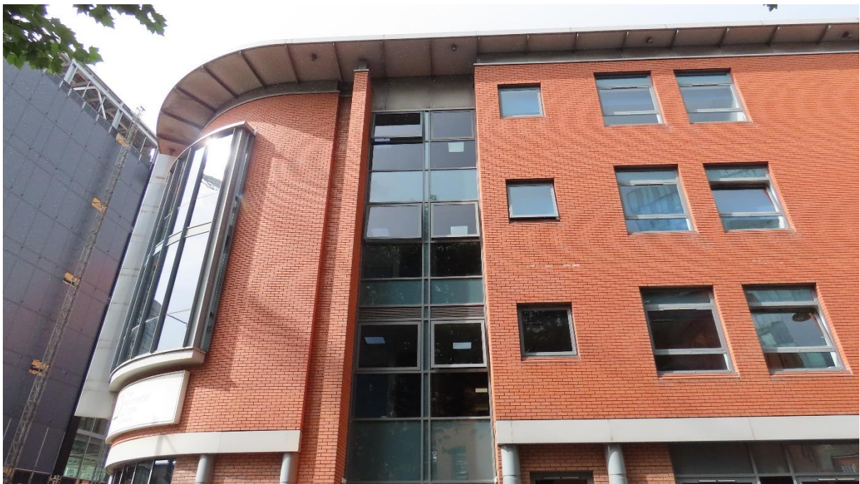
Photograph 2: The southern corner of the south-east aspect of the building
