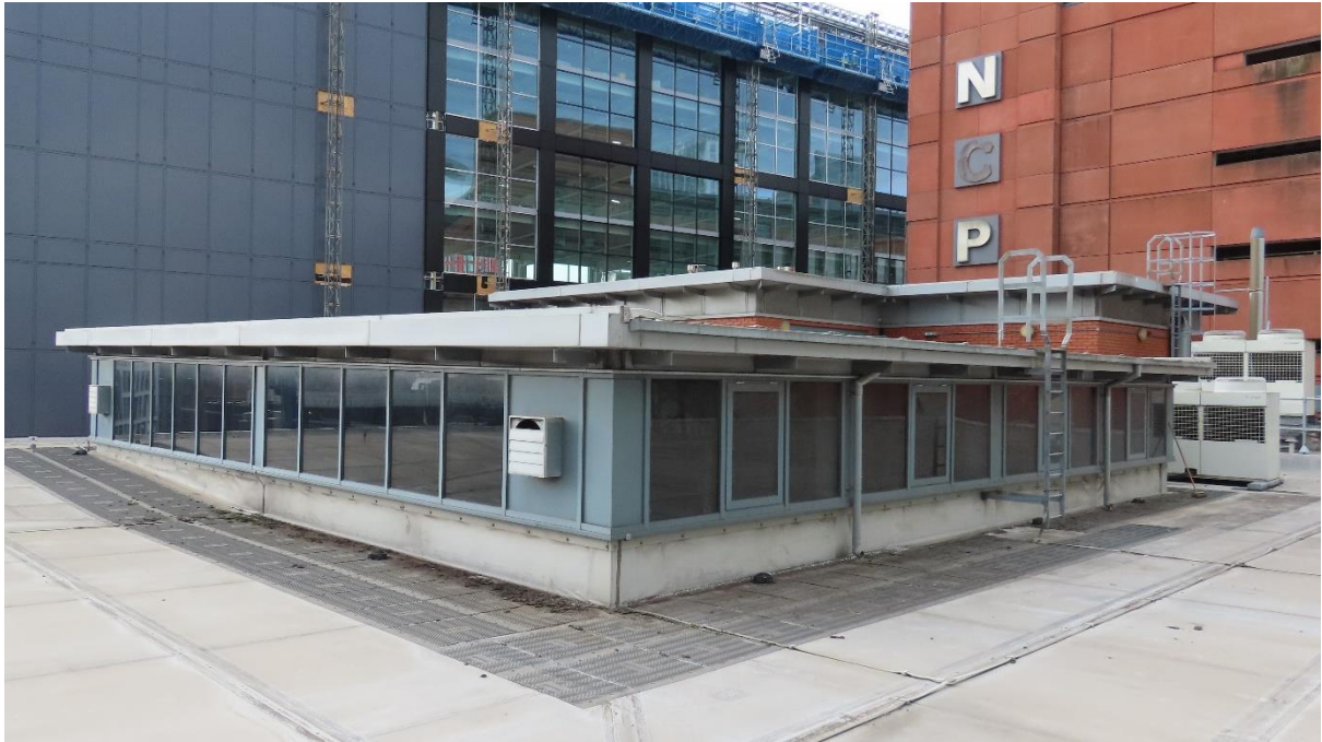
Photograph 5: The rooftop of the building
