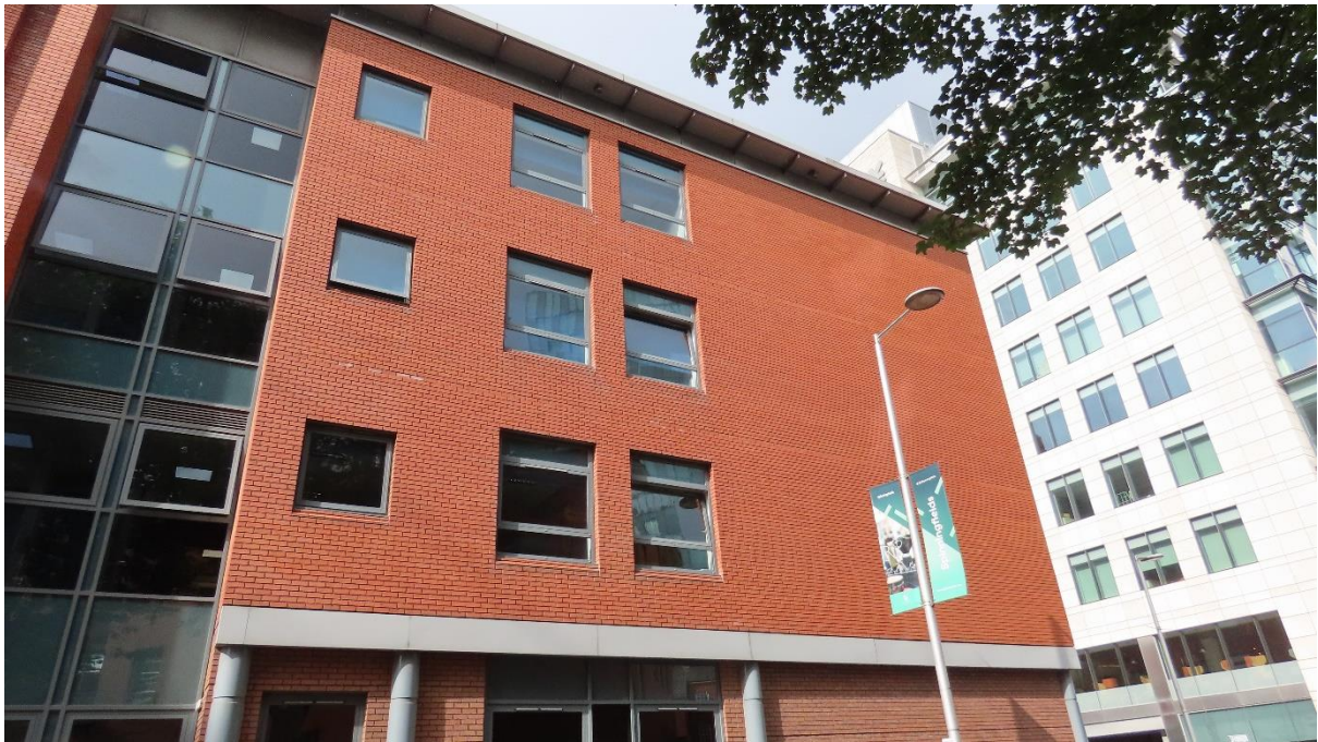
Photograph 3: The northern corner of the south-east aspect of the building
