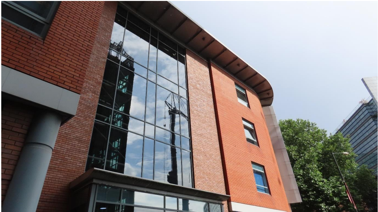
Photograph 1: The south-west aspect of the building
