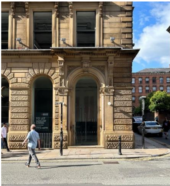
Figure 1: Existing Peter Street Entrance
