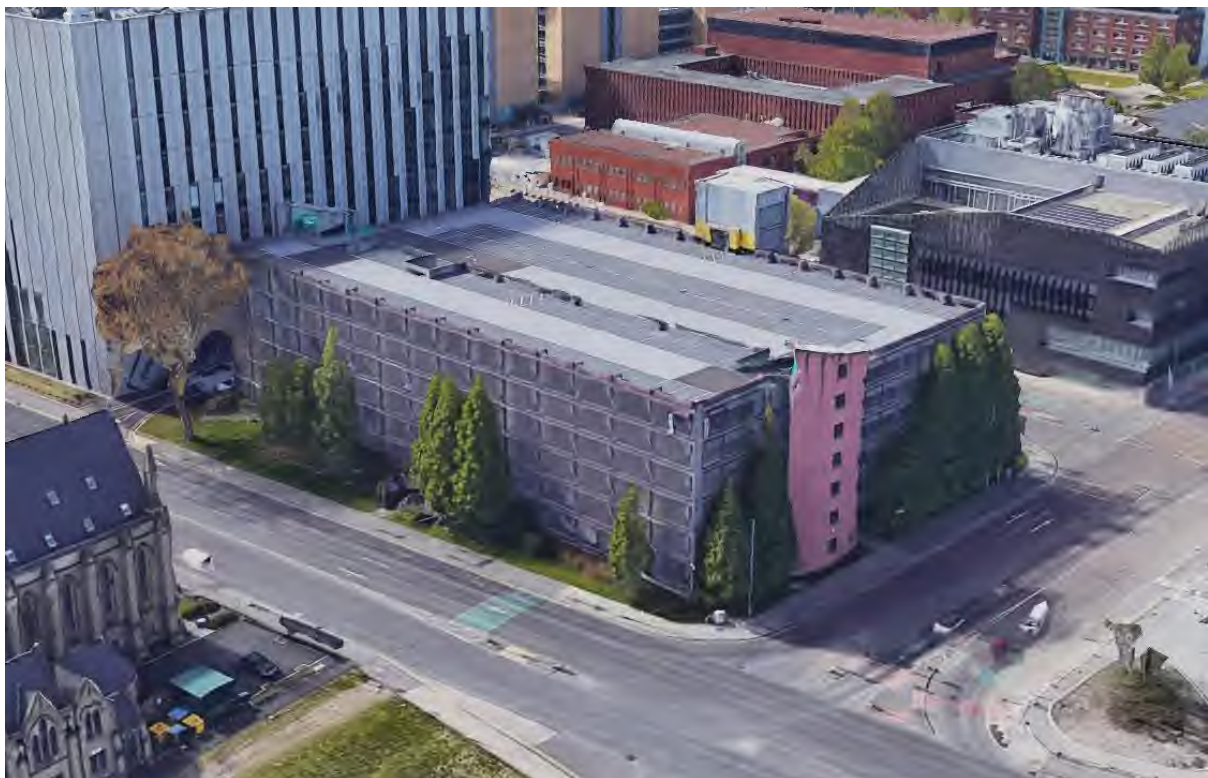
Figure 15 – Multistorey Aquatics Centre car park
