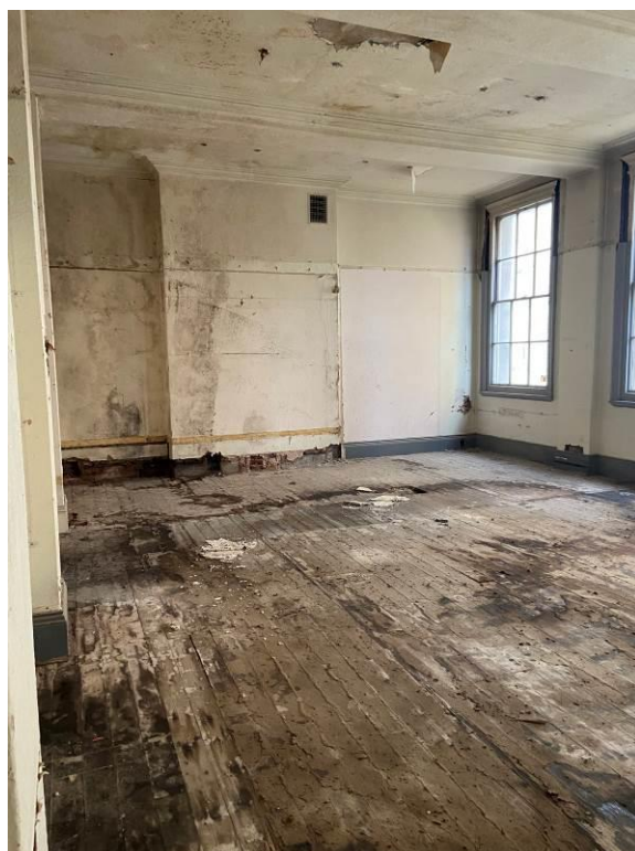
Figure 29: Large room at upper level.
