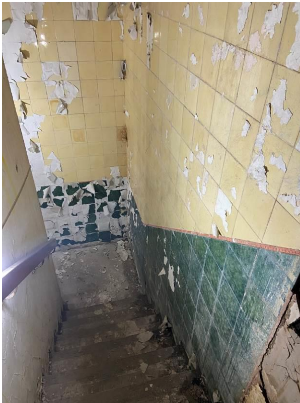
Figure 20: Tiled staircase leading to the basement from the ground floor.
