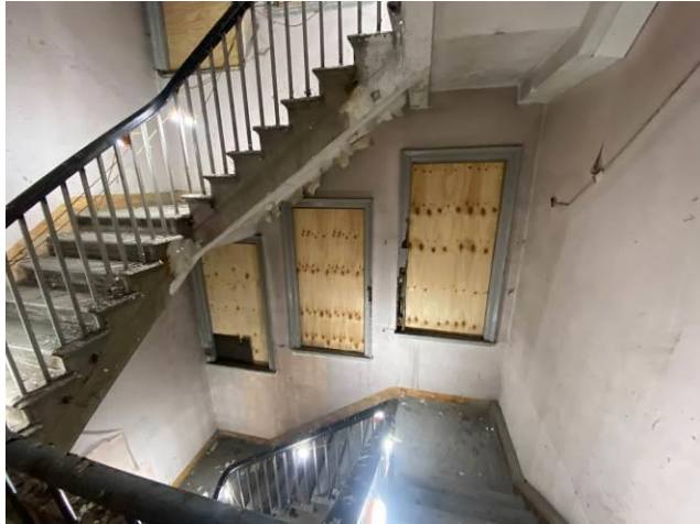
Figure 30: Tiered windows in stair core.
