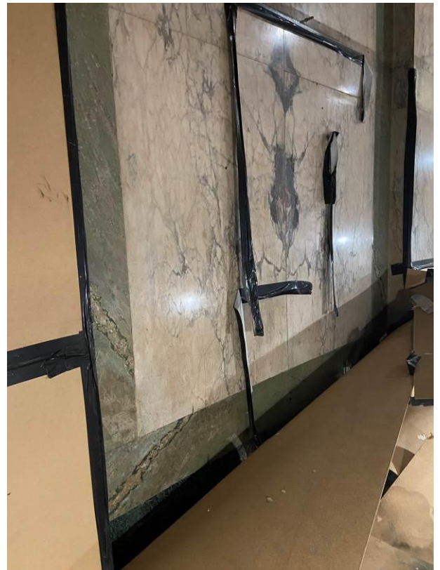
Figure 21: Marble panels in entrance corridor from the ground floor.
