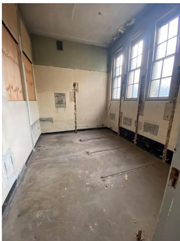
Figure 28: Former toilet block.
