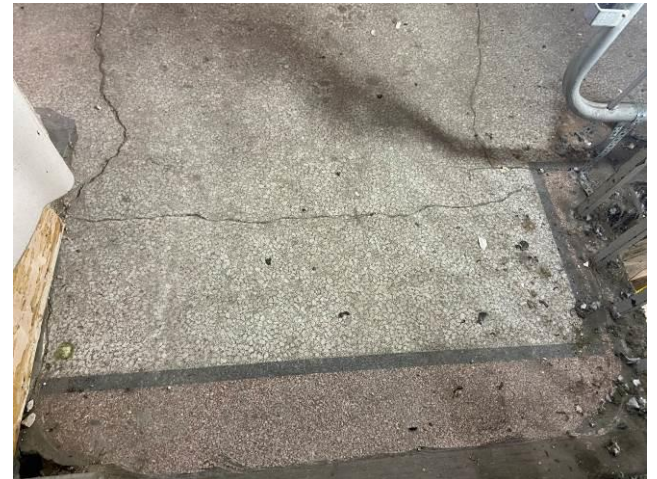
Figure 33: Terrazzo floor in upstairs corridors.
