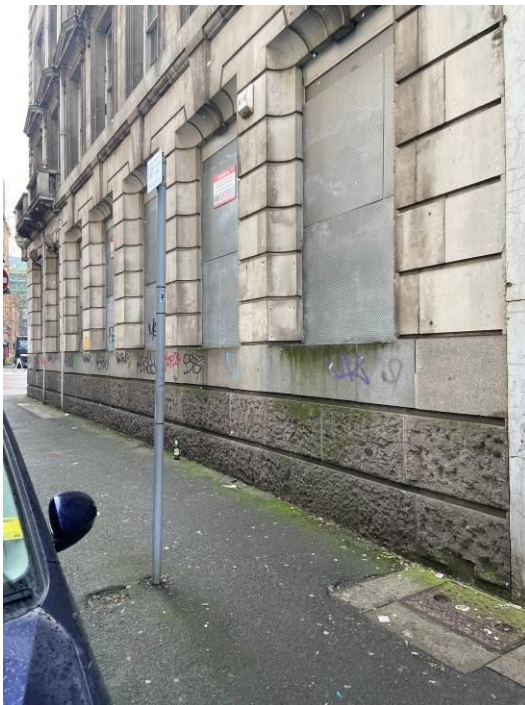
Figure 16: Chatham Street elevation with temporary grilles in place to protect windows.
