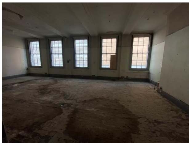
Figure 27: Large room at upper level.
