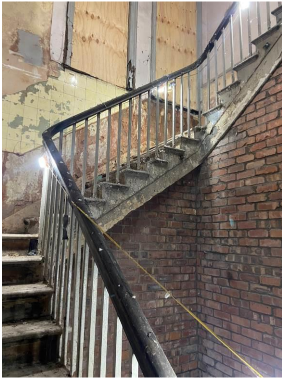
Figure 22: Utilitarian main stair which extends all the way up the building and formerly wrapped around a lift.
