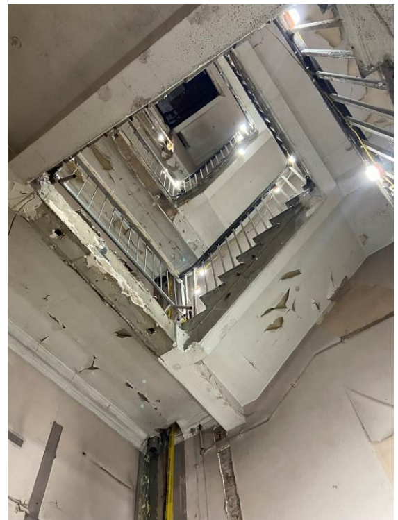
Figure 23: Extension of main stair upwards through the building and central well.
