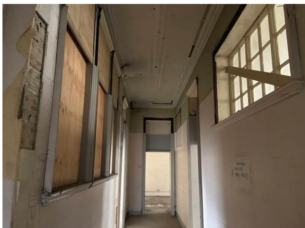
Figure 26: Corridor at upper level with interior windows.
