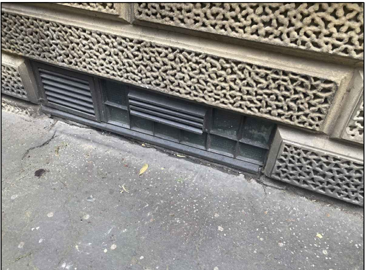
PHOTO 1 - EXISTING VENTS ON CHANCERY LANE
