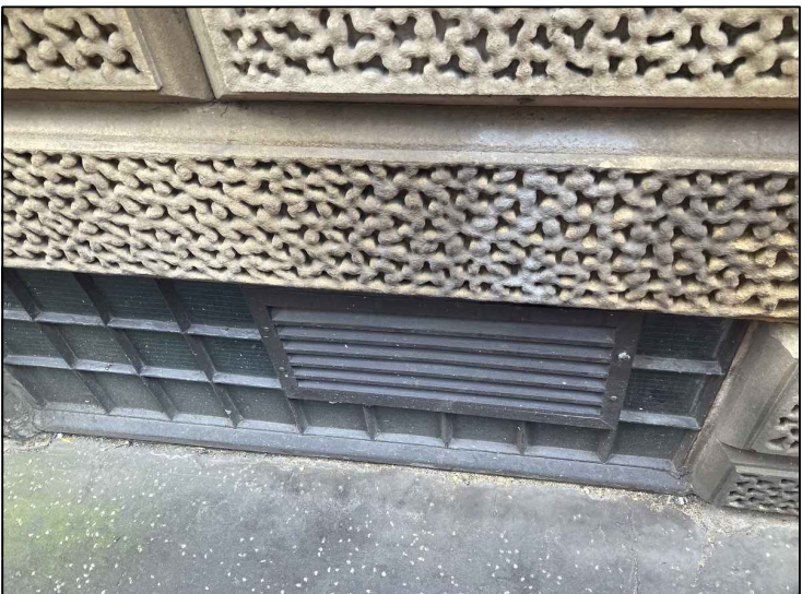
PHOTO 3 - EXISTING VENTS ON CHANCERY LANE
