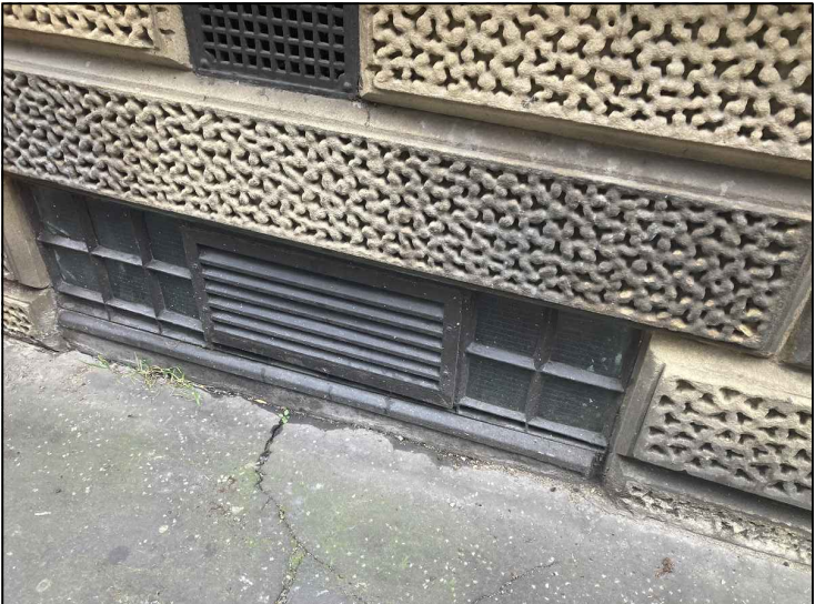
PHOTO 2 - EXISTING VENTS ON CHANCERY LANE
