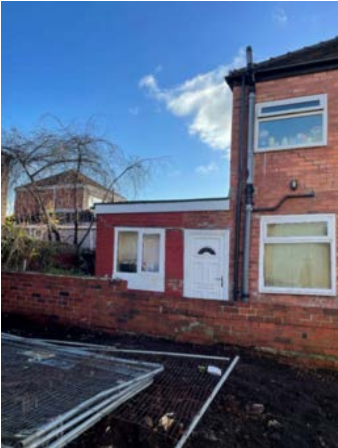
Photograph 5: Facing south towards adjacent property
