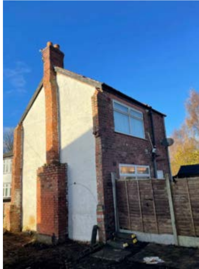
Photograph 4: Facing north-west towards adjacent property
