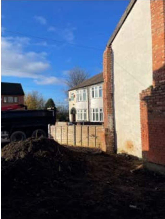
Photograph 3: Western part of the Site - looking north-west towards adjacent property
