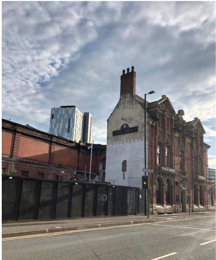
Plate 3 View of eastern elevation of the Star and Garter from Fairfield Road
