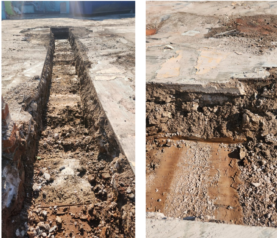
Figure 3 Photographs of Existing Clay Ground Conditions
