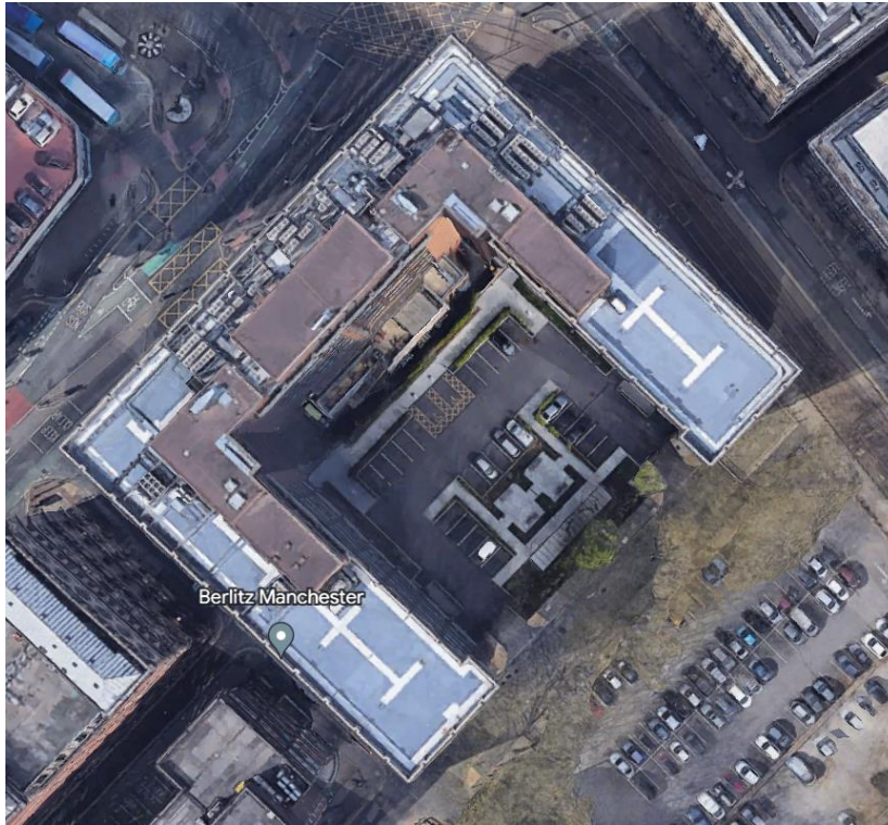
Typical Location of existing Mechanical Plant
