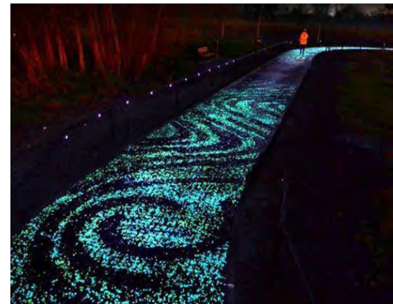
5. Tarmac with luminescent chippings
