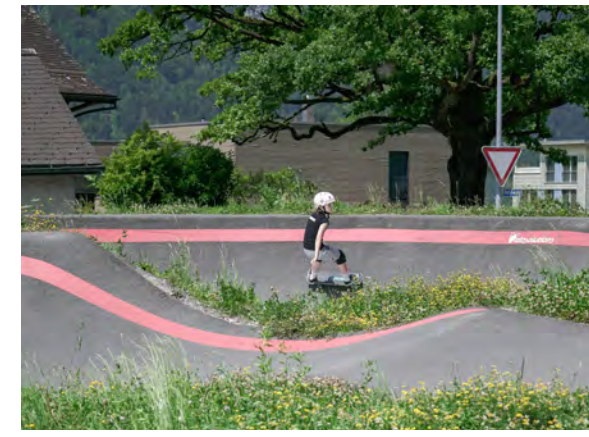
3. Asphalt track with thermoplastic markings
