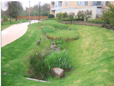
Track drains to planted sustainable swale
