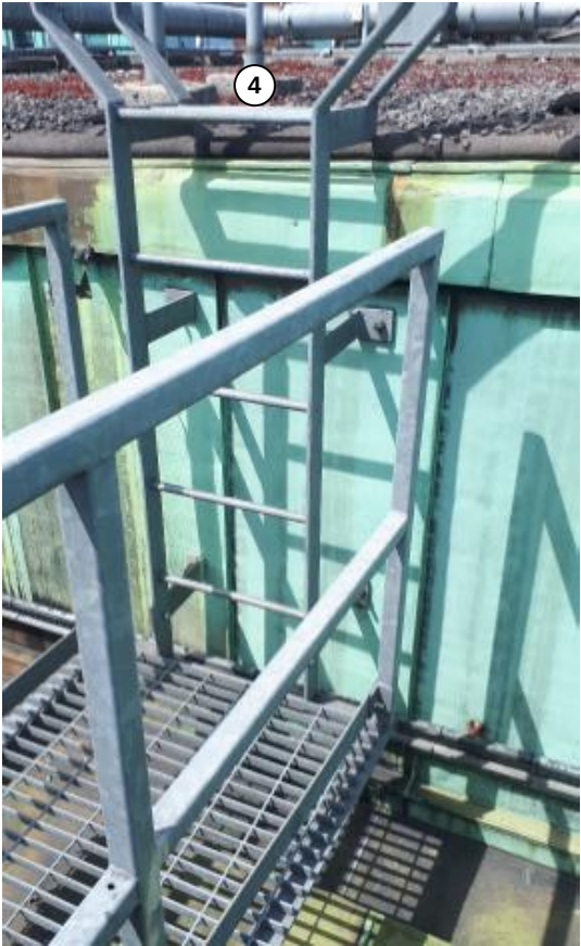
Figure 5 - Access to plant roof area
