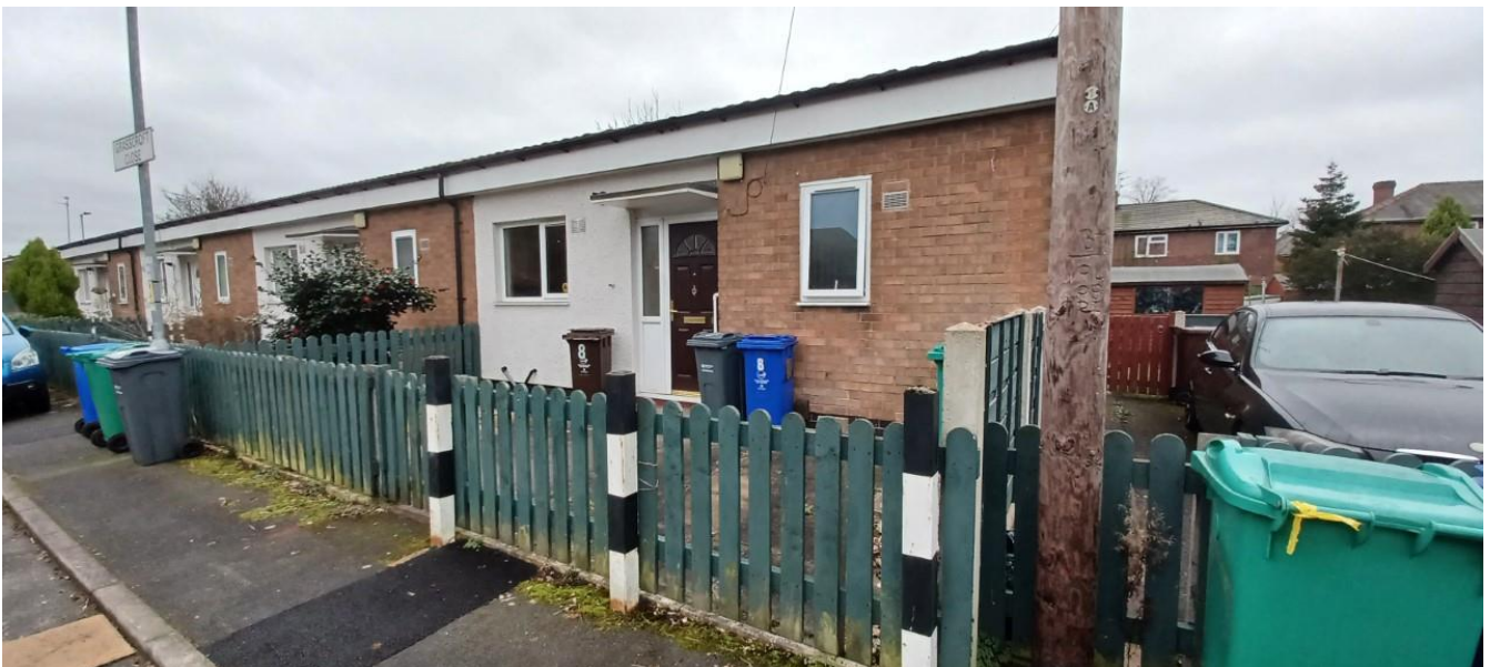
Figure 1. Principal elevation of the property.
