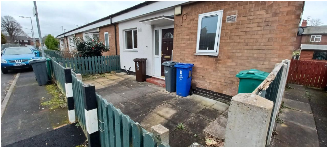
Figure 2. Existing paved area located to the front of the property.
