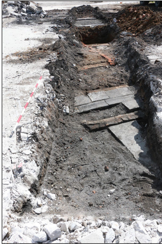
Plate 17: General shot of Trench 6 showing 19 th century remains, looking east. Scale = 1 x 2m.
