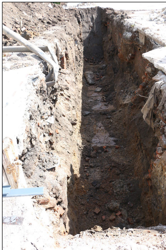
Plate 8: General shot of Trench 3 after the 19 th century remains were removed, looking north-east. Scale = 1 x 2m.
