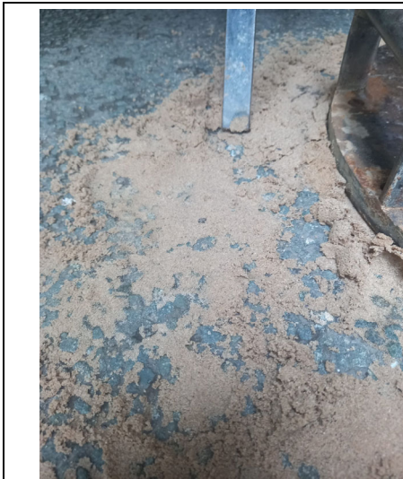
Photograph of Material Tested
