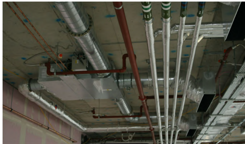
Figure. 5.5.2 - Typical 4-pipe Fan Coil Unit Installation
